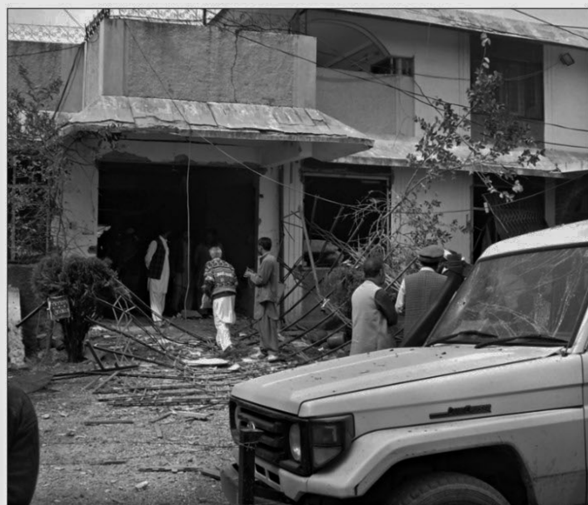
Pakistani security officials inspect a damaged building of a US-based Christian charity after a militant attack near the town of Oghi in the Mansehra district of North West Frontier Province (NWFP) yesterday. Militants armed with guns and grenades stormed the offices of a US-based Christian charity in Pakistan, killing six aid workers in an attack blamed on Islamist rebels.
