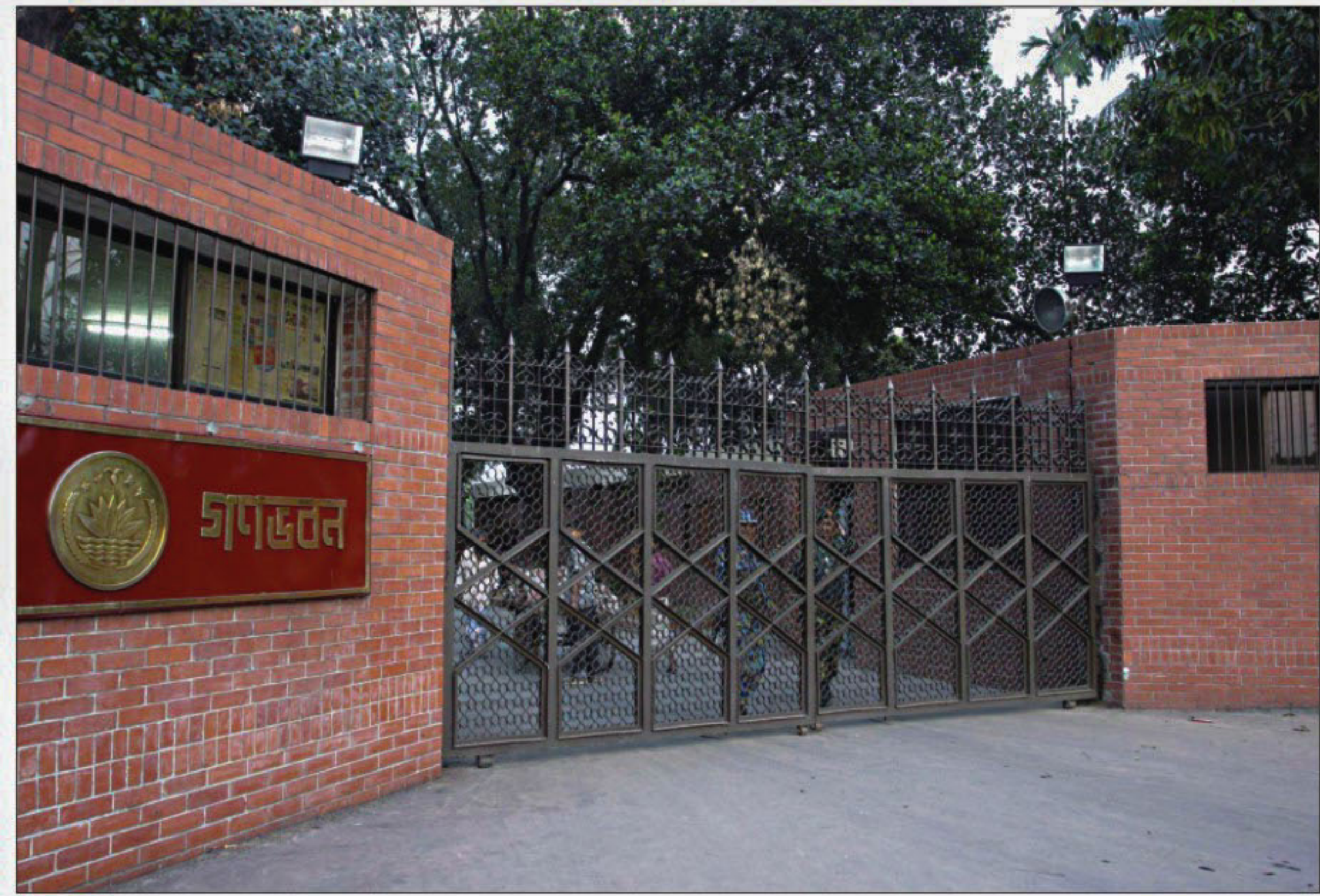
Gono Bhaban—official residence of the prime minister. Sheikh Hasina has moved here after living in state guesthouse Jamuna for a little over a year. PHOTO: STAR
