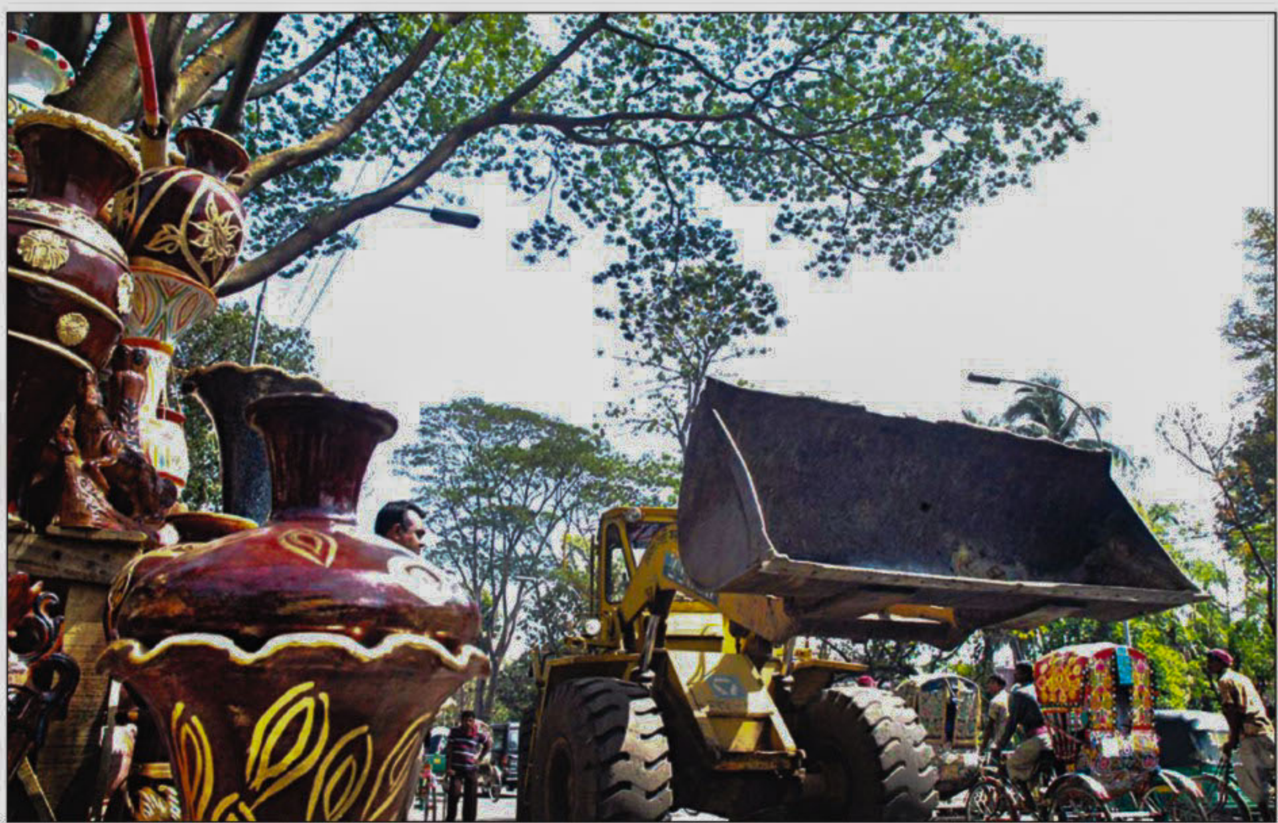
Dhaka City Corporation launches an eviction drive against the illegal structures erected on the footpath in front of Bangladesh Shishu Academy in the city yesterday. Vendors used the footpath to sell colourful earthenware.
