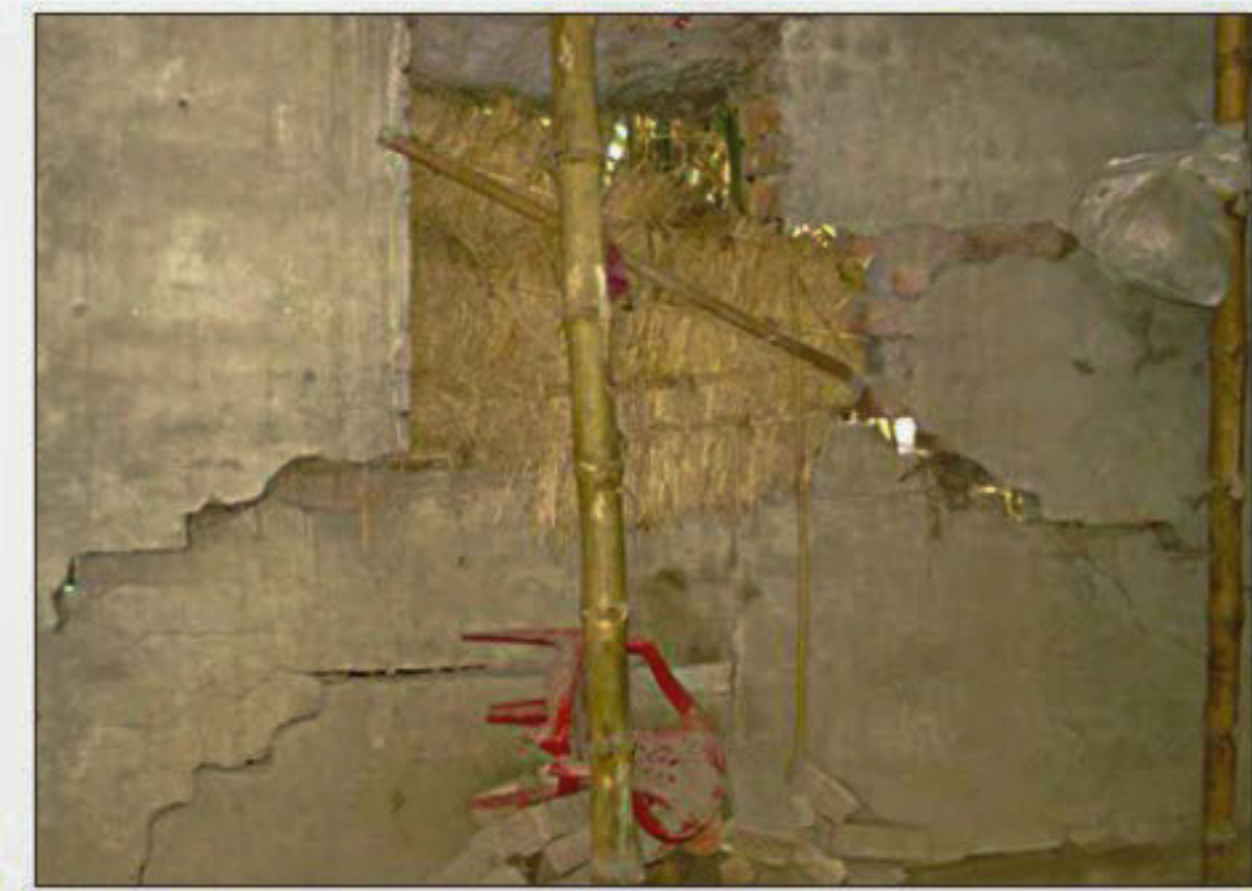
Cracks developed at the house of Aftab Uddin at Gigagari village under Parbatipur upazila of Dinajpur district, right, a classroom of Kaderia Dimukhi Dakhil Madrasa at Barapukuria village under Parbatipur upazila of Dinajpur collapsed due to the impact of land subsidence around Barapukuria coalmine.
