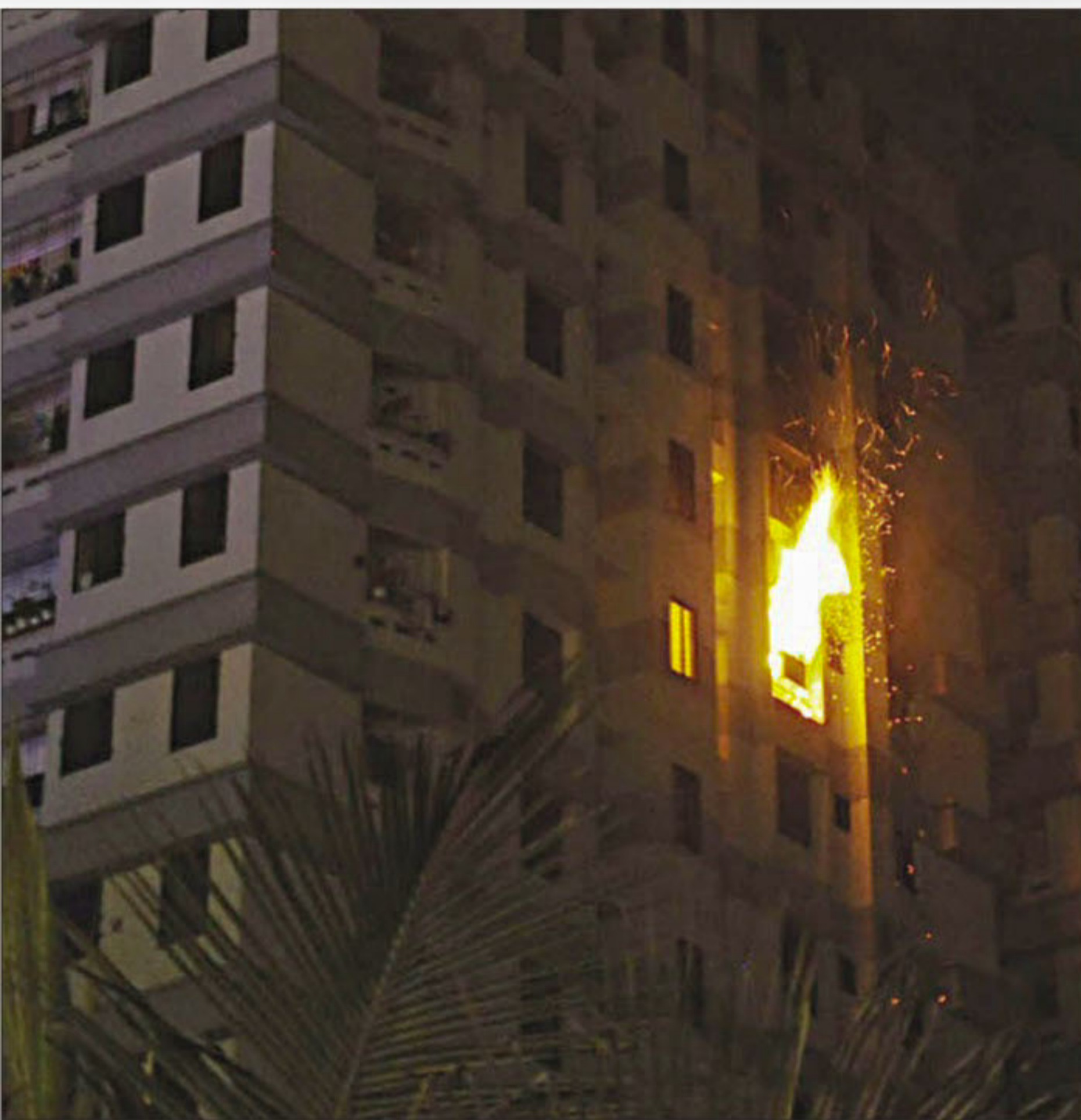
(Clockwise from left) Flames come out of an apartment on the 10th floor of Japan Garden City as a fire broke out on Thursday night. Neighbours console a relative of the victims who died in the fire. Materials for interior decoration and equipment were gutted in the flat.
