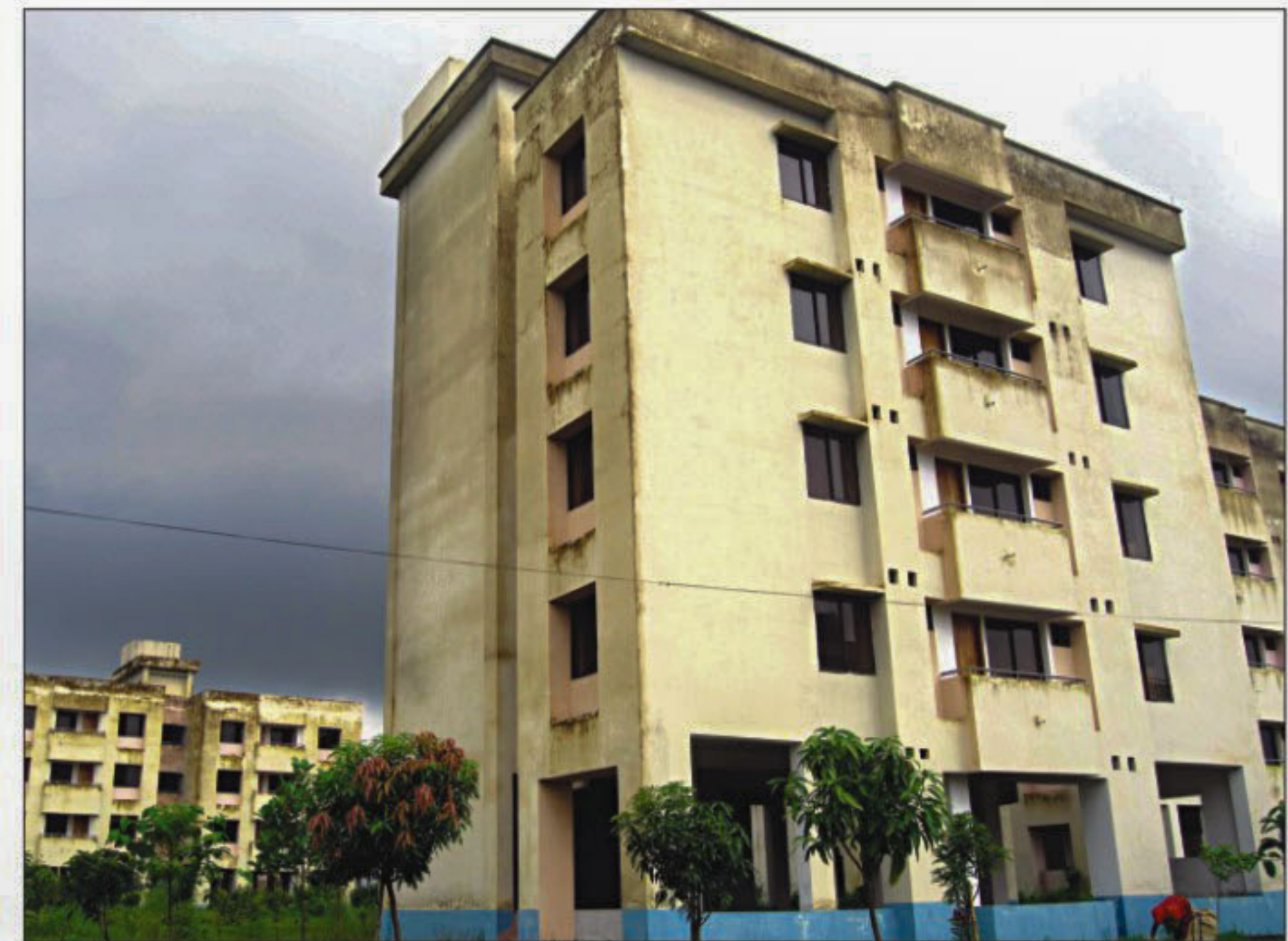
A large number of unused staff quarters, built for doctors of Shaheed Ziaur Rahman Medical College and Hospital in Bogra town about four years ago, remain as a burden for the authorities as the allottees stay at rented houses in the town.
