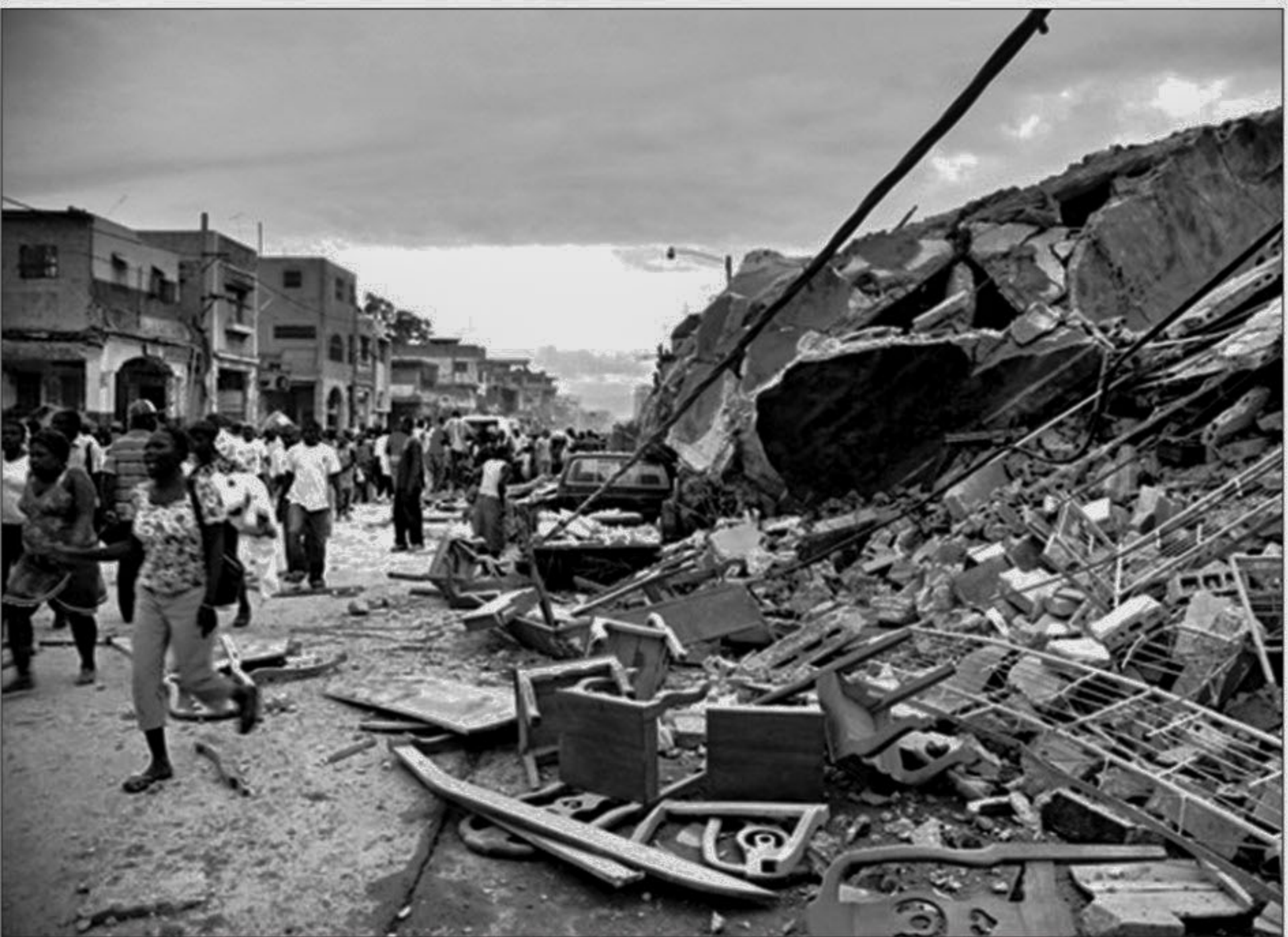
Haitians walk past damaged structures on Tuesday in capital Port-au-Prince after a huge earthquake measuring 7.0 rocked the impoverished Caribbean country, toppling buildings and causing widespread damage and panic.
