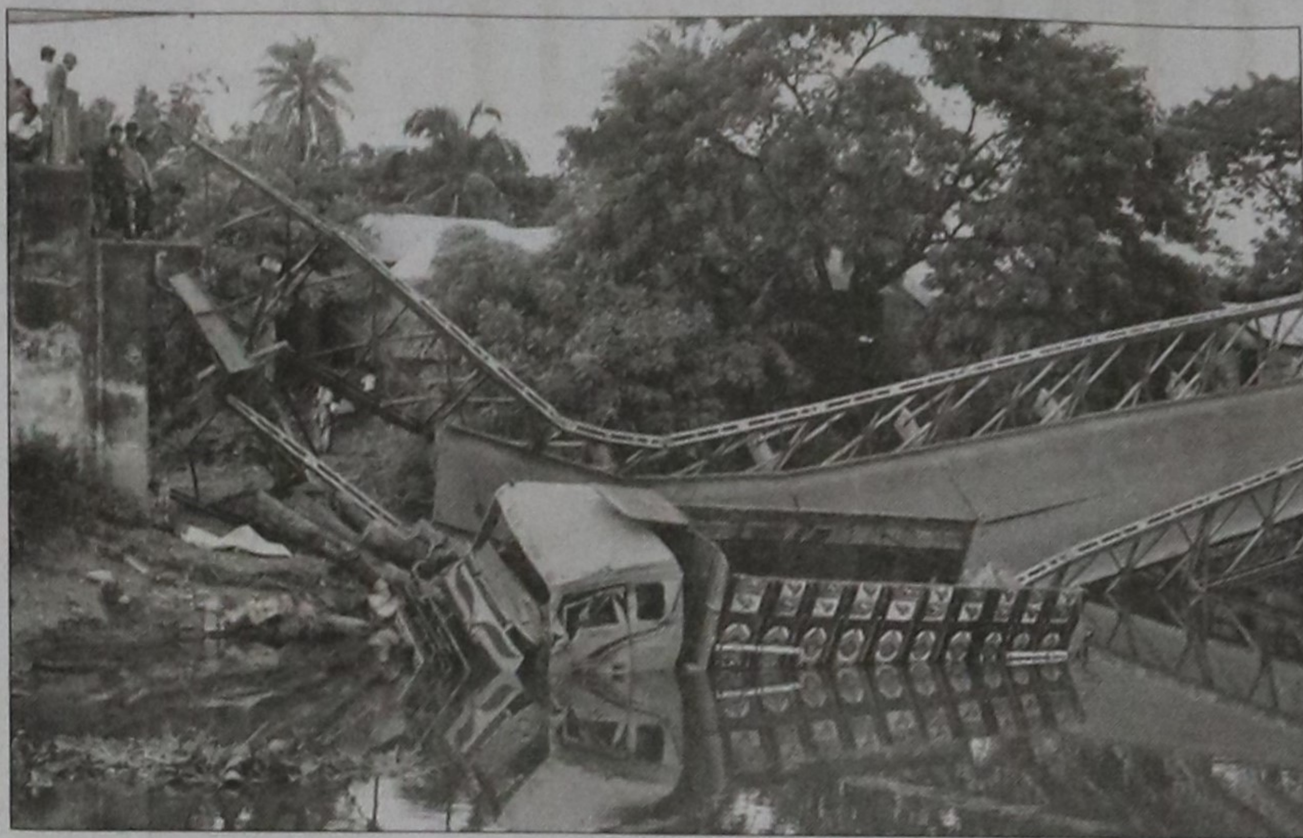
A goods-laden truck falls into a water body as the steel-made bailey bridge in Bhumi area on Singair-Gabtol road in Manikganj collapsed under the weight of the truck yesterday. However, there was no report of casualties.
