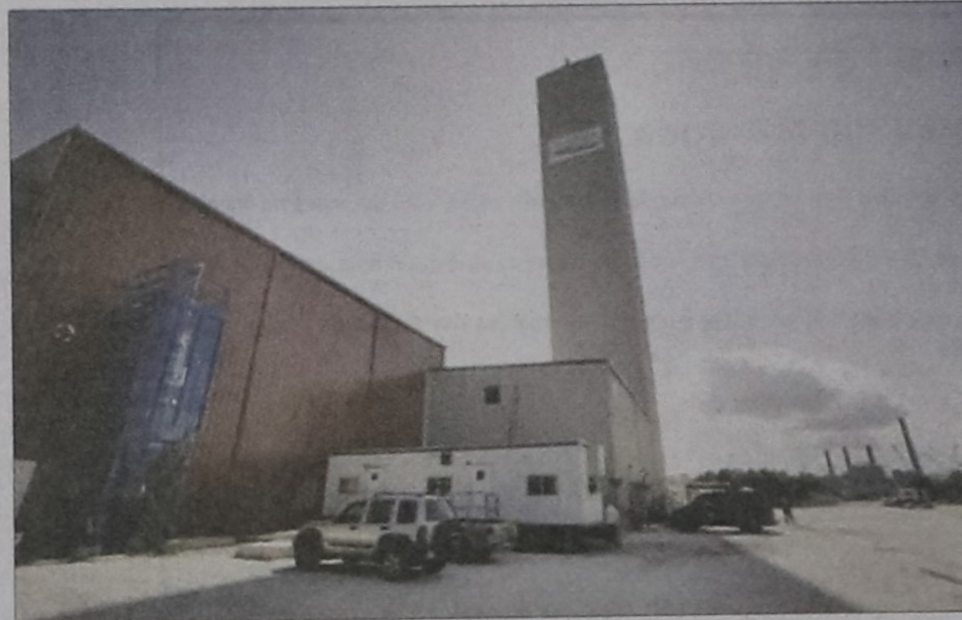
In this photo made on September 29, a 20-storey tower housing a reactor, which converts coal into natural gas, carbon dioxide and hydrogen, is seen at the GreatPoint Energy test facility in Somerset, Massachusetts. GreatPoint Energy has developed a technique for turning coal into natural gas more cheaply and efficiently than previous methods.
