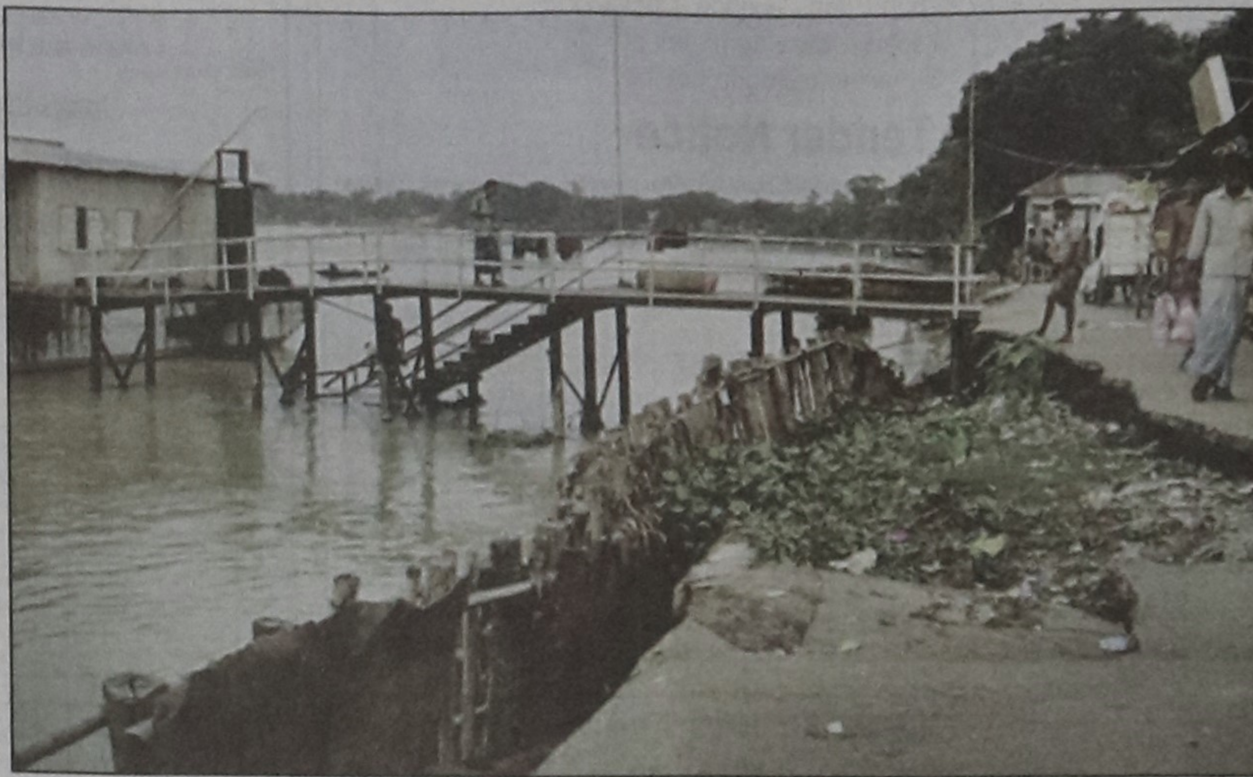
Erosion of the road connecting the bridge leading to the pontoon of launch terminal in Sunamganj town makes the place vulnerable to accident anytime.
