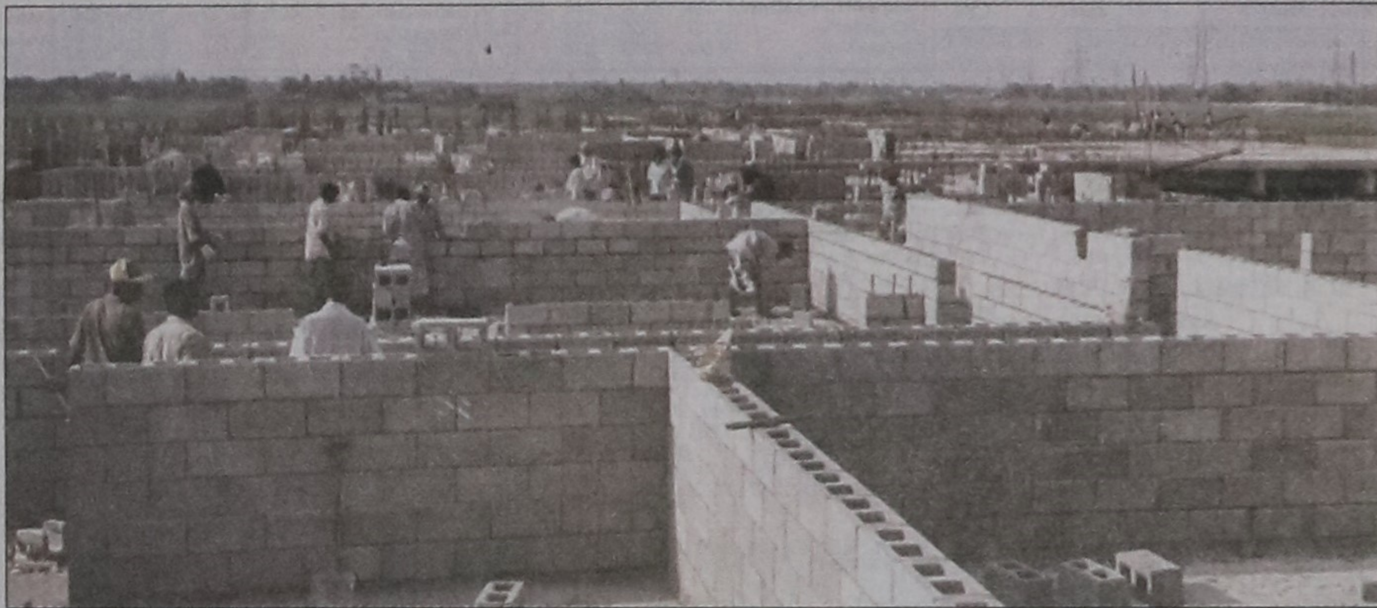
Workers use hollow blocks at a construction site in Dhaka.
