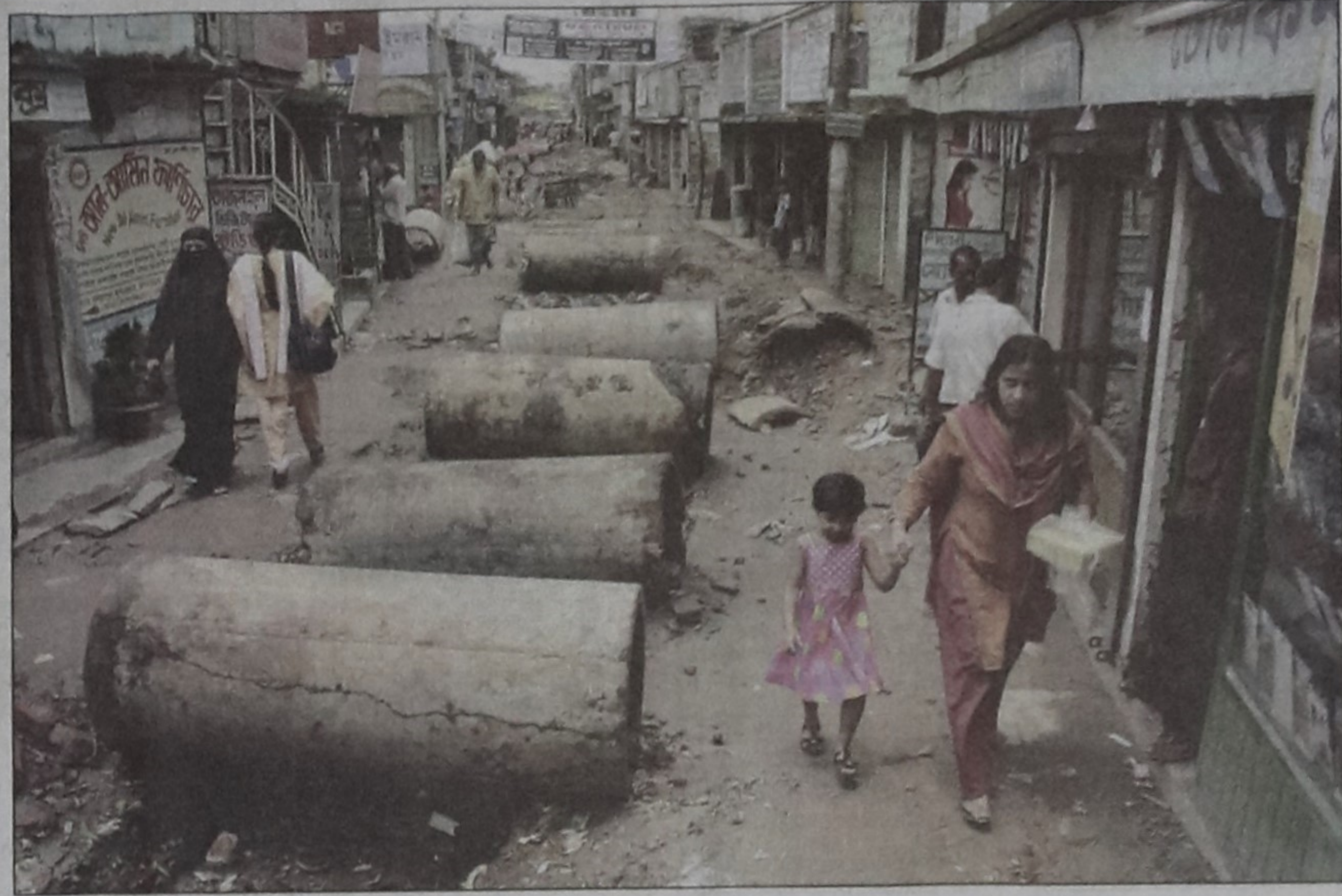
The road at Kalyanpur Naton Bazar lies in dilapidated condition for long, causing immense suffering to the locals. The photo was taken yesterday.
