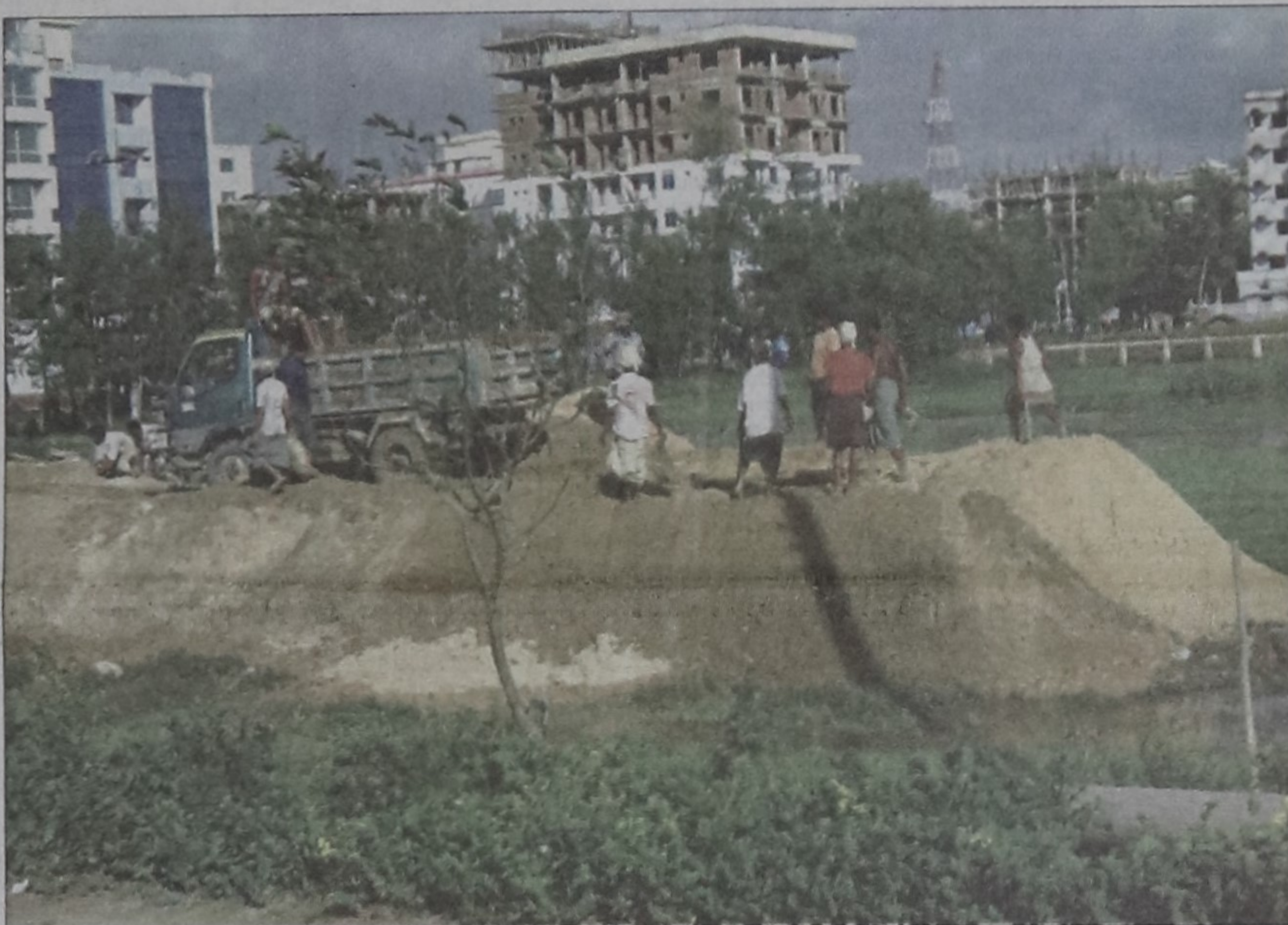
A low, flat land inside Cox's Bazar hotel-motel zone is being filled with earth moved from hills.
