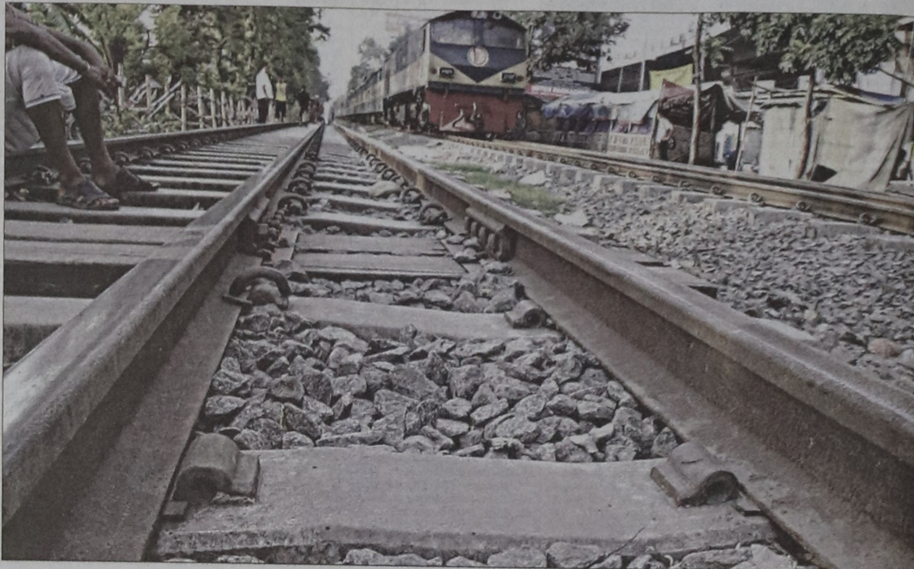
This photo taken near Mohakhali level crossing shows a number of the clips, which hold the rails to the sleepers, are missing. Locals claim addicts who spend time there at night stole the clips a few days ago. The authorities appear to be oblivious to the missing clips.
