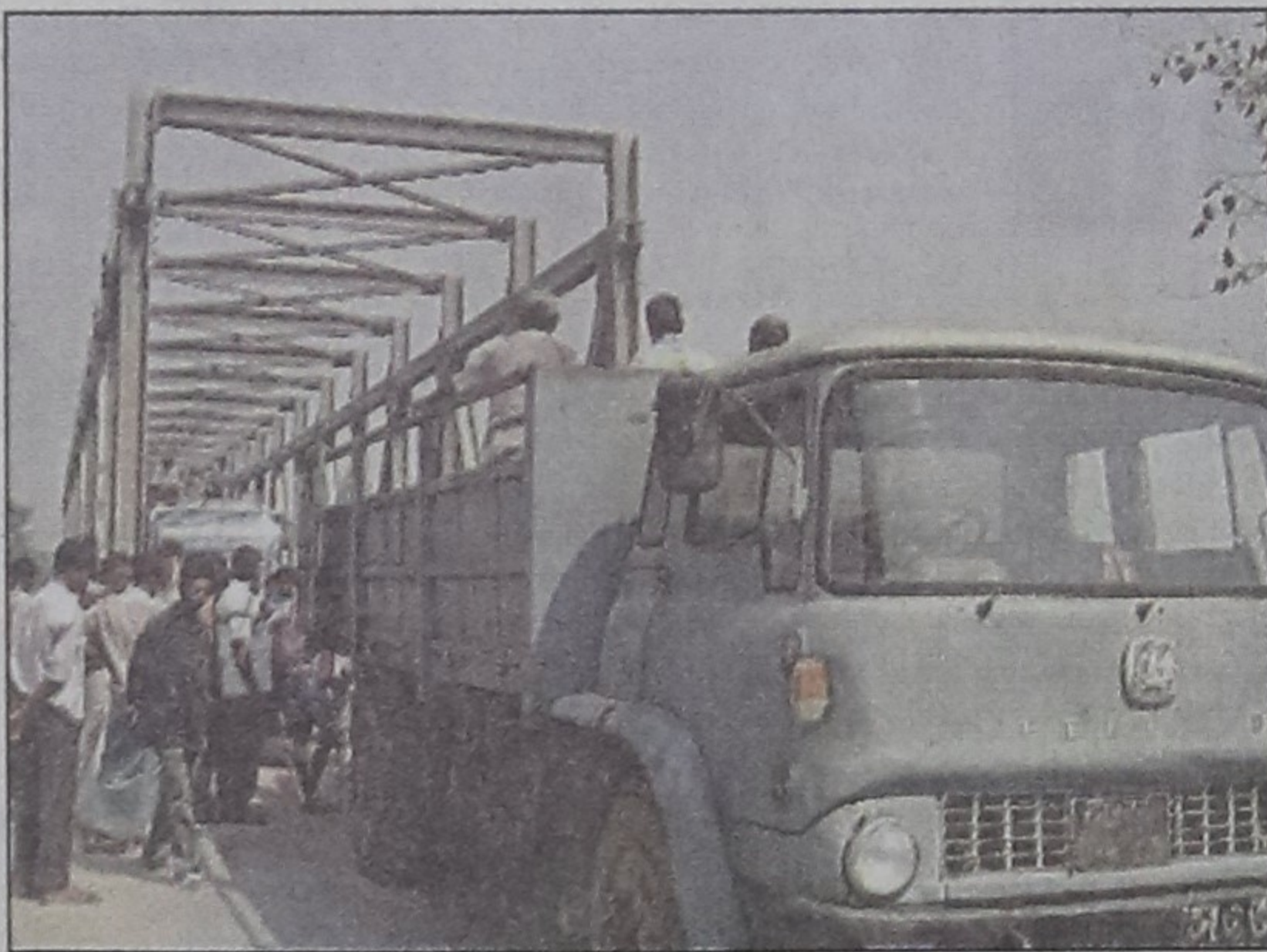
RISKY DRIVE: These two awfully dilapidated bailey bridges, one at Sakoa of Gaibandha-Palashbari road, left, and the other at Badiakhali Bazar of Gaibandha-Fulchhari road, are among at least six such structures in Gaibandha. The bridges, set as temporary substitute for the concrete ones several years ago, still await replacement.
