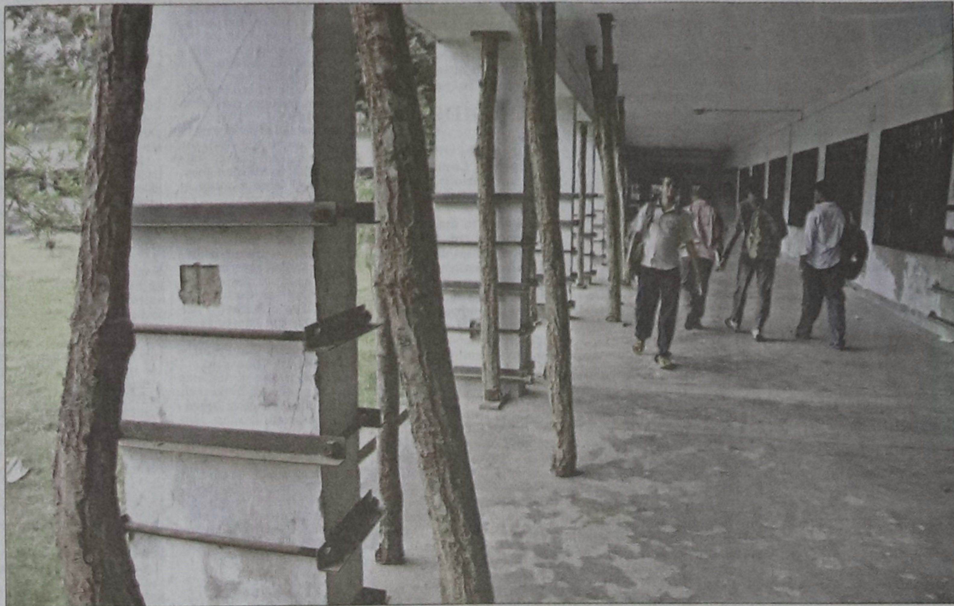
Authorities have recently installed iron braces around pillars in one portion of the Mohsin Hall at Dhaka University to prevent the roofs from collapsing. They had earlier propped up the ceilings with wooden logs after the roofs developed several cracks. Several thousand students now live in the dormitory risking their lives.
