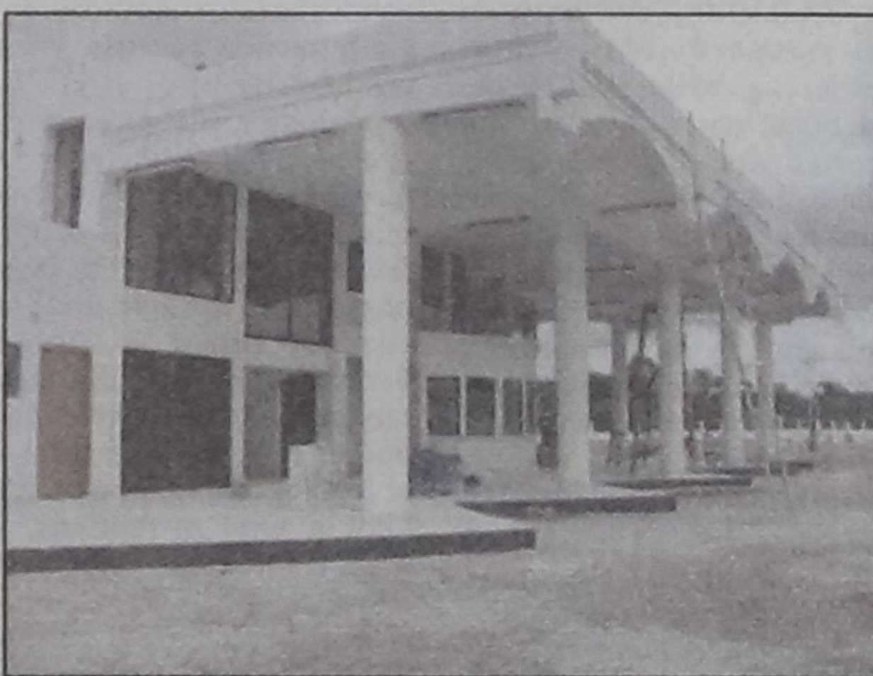
New building of Patuakhali central bus terminal, constructed at a cost of Tk 3.51 crore on three acres of land in the town's Kalikapur area, was opened yesterday. PHOTO: STAR
