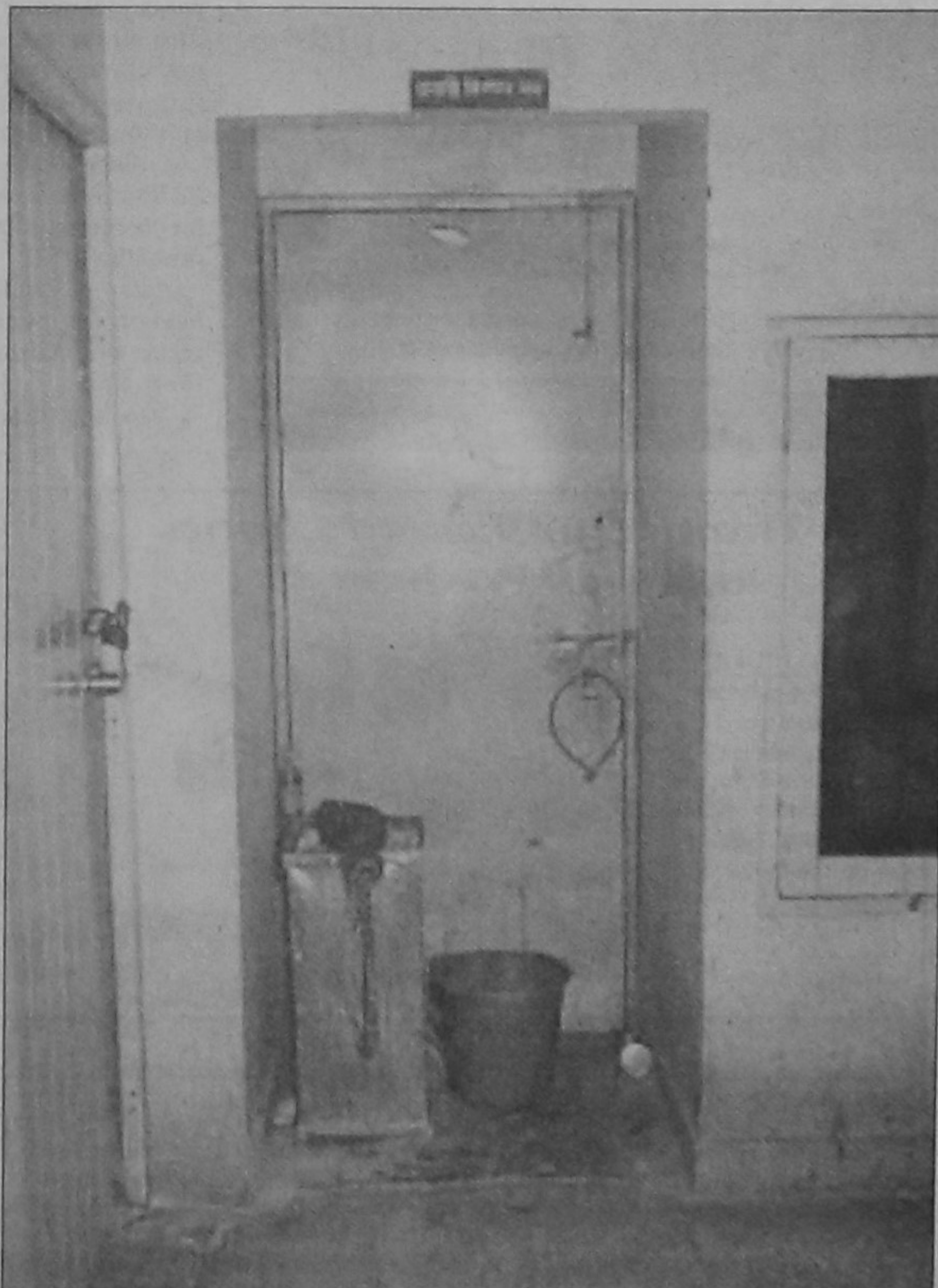
Figure 6: Useless Fire Escape at Dilkusha's BCIC Bhaban, as the final door is locked from outside it.
