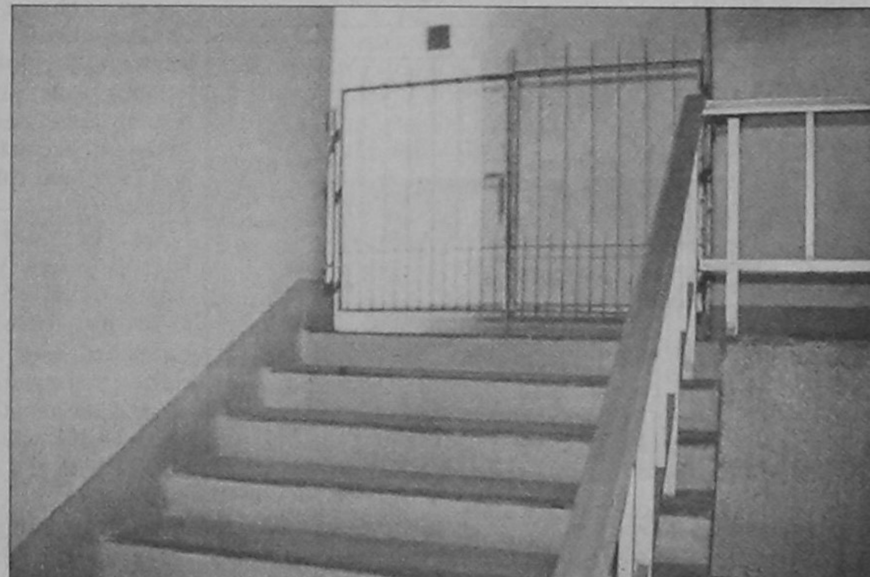
Figure 5: Barricaded staircases. This one is on the 14th floor of 20-storied BSB Building on RAJUK Avenue taken some years back. Today there is a floor-to-ceiling fencing in addition.
