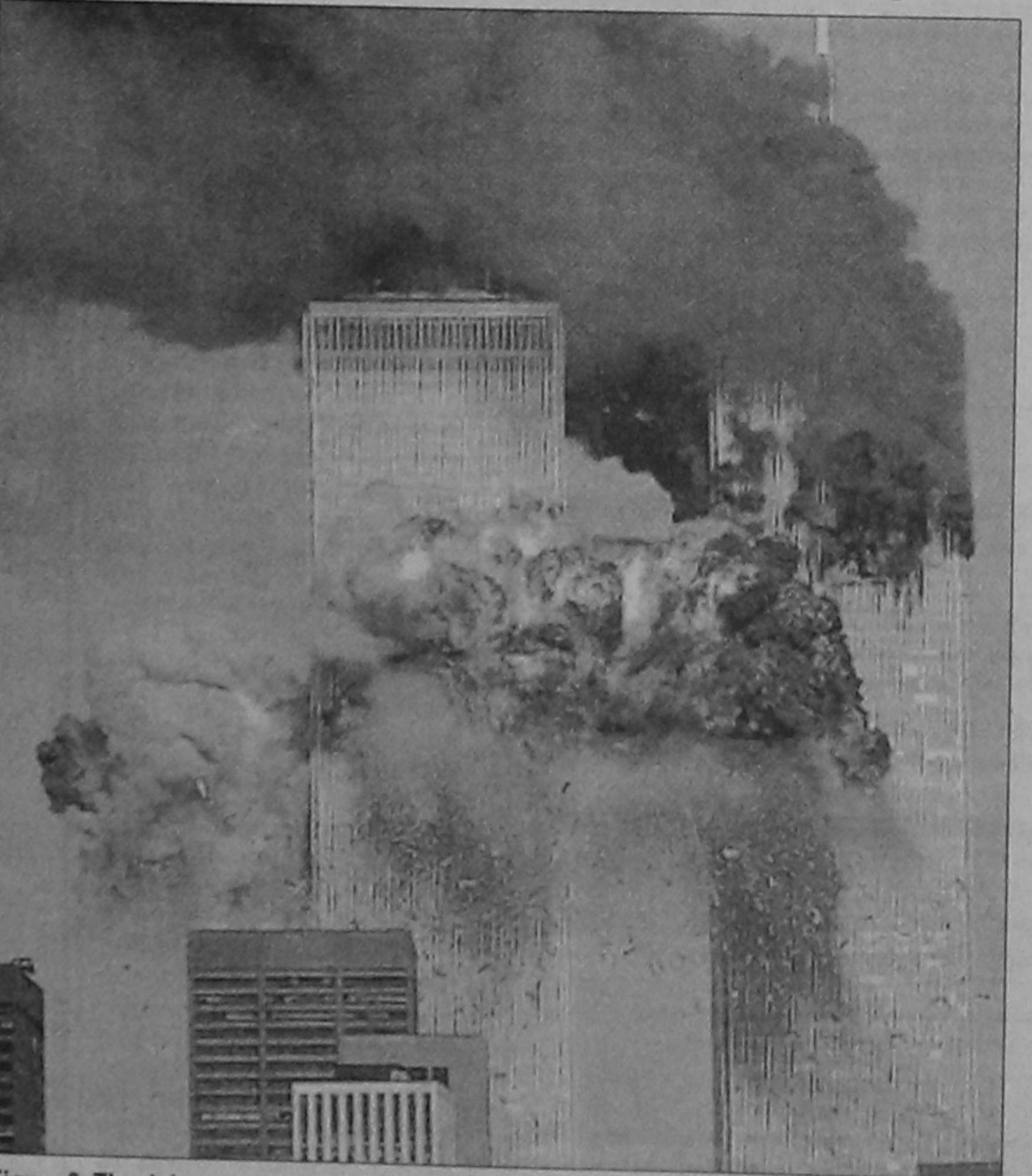
Figure 3: The dying moments of the Twin Towers before its 9/11 collapse
