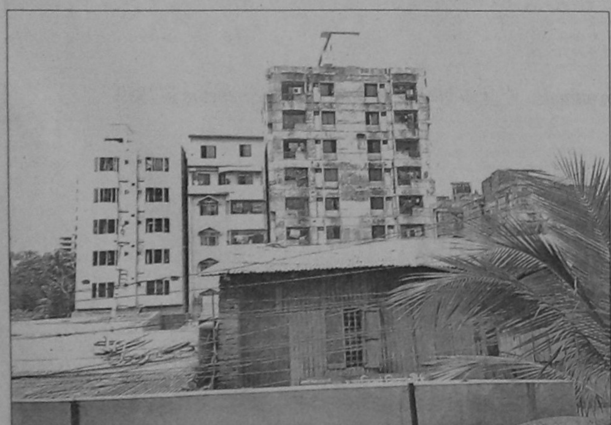
Figure 1 Buildings constructed under the 1996 rules defy rhyme, reason or logic
