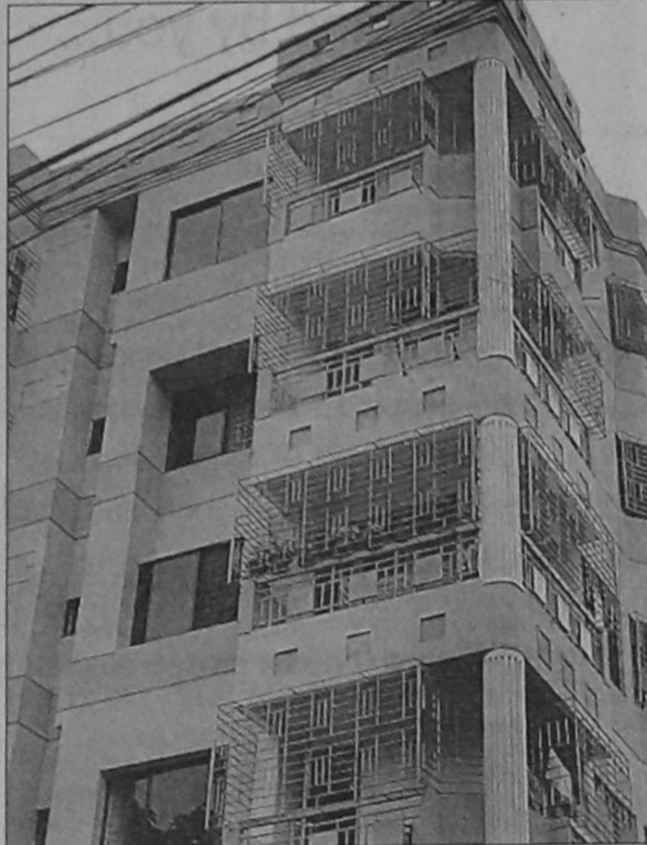
Figure 2 Extensive but essential security measures by fixed grille may make buildings unsafe in a fire by preventing exit. Such grille may be made partly operable for safety of inmates.
