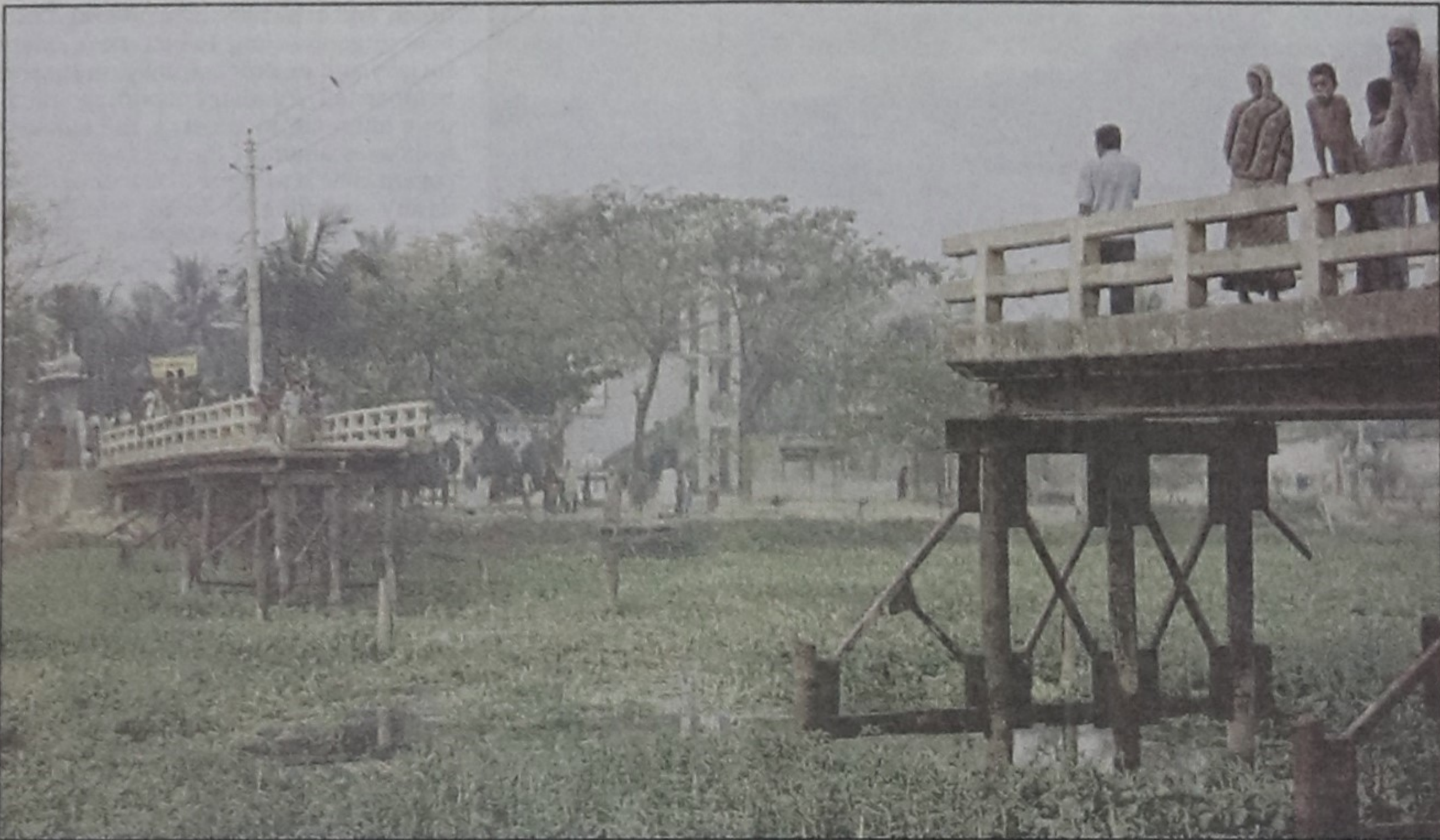
Hardly 12 years into opening, middle portion of the bridge across Mayur River near Khulna city collapsed on Wednesday, much to the sufferings of commuters from Khulna city to Satkhira. Substandard materials were allegedly used for construction of the bridge.
