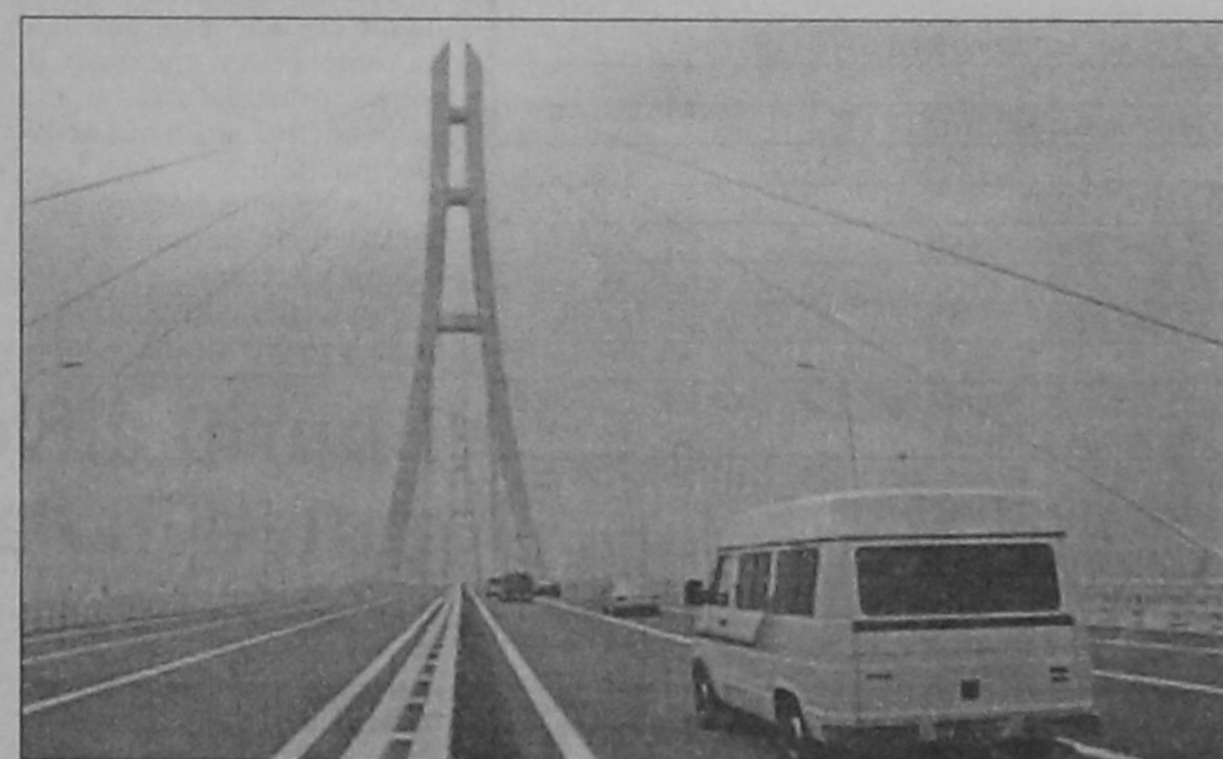
Yangtze River Cable-Stayed Highway Bridge, an example of Chinese technology.
