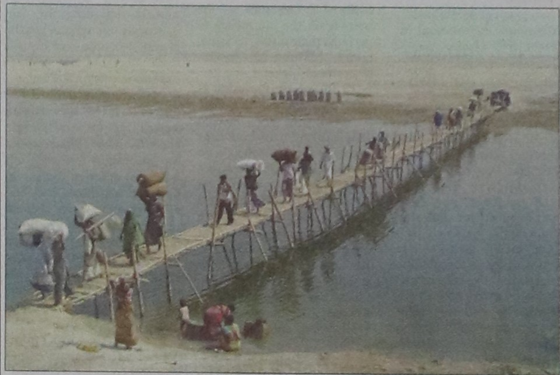
People of char areas in Fulchhari upazila under Gaibandha district have constructed this hundred-yard-long bamboo bridge across a tributary of the Jamuna on self-help basis.
