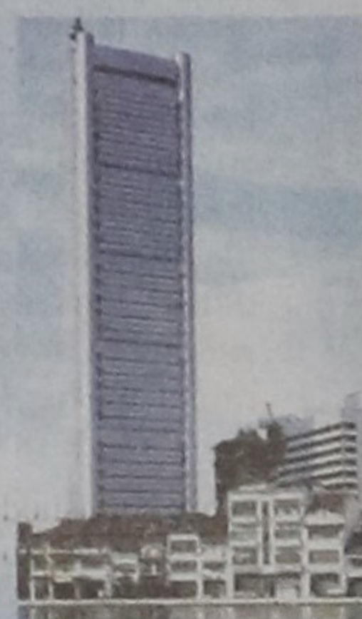
Telecom Building in Singapore
