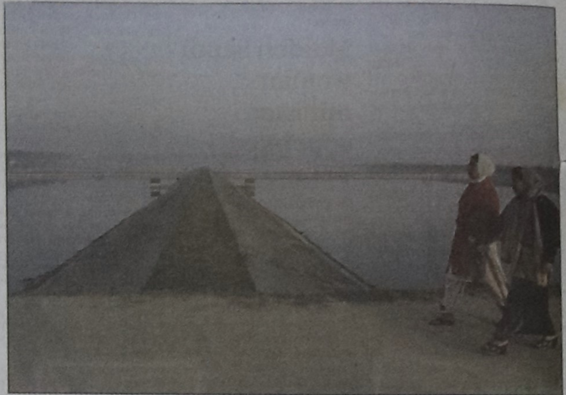
These lagoons of Dhaka Wasa's Sewerage Treatment Plant in Pagla, Narayanganj, have plenty of fish in them which criminals catch and sell in nearby markets caring little about the buyers' health.
