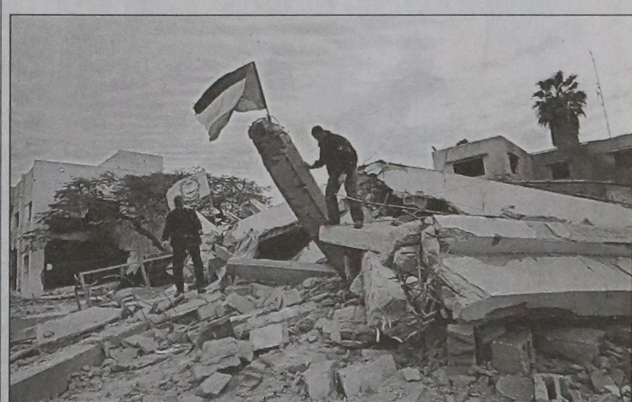
Palestinian security men inspect the damage at a police post targeted by an Israeli air raid early yesterday near Khan Yunis in the southern Gaza strip. An Israeli F-16 fired two missiles against the police post, causing material damage but no injuries, witnesses and Palestinian security sources said.
