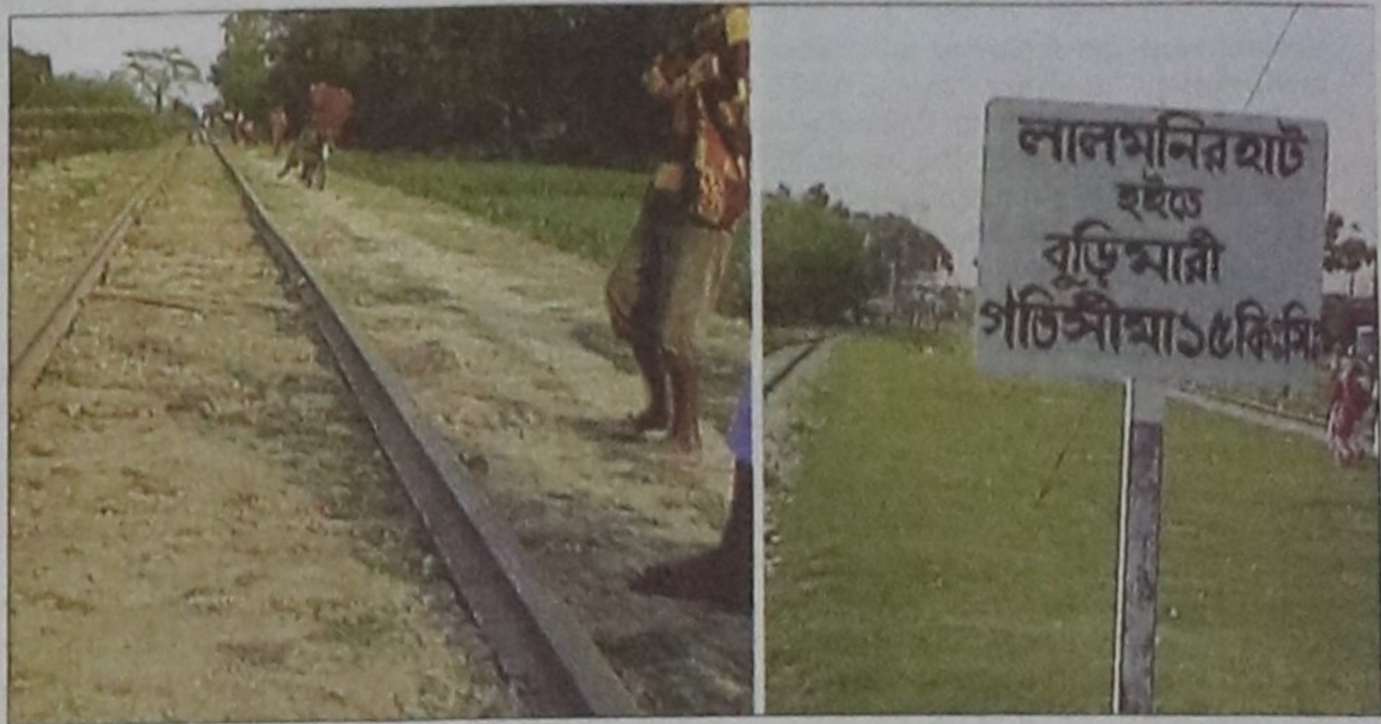
A railway track without sleepers and stones near Aditmari station on Lalmonirhat-Burimari line, left, and a Bangladesh Railway signpost indicating 15 km per hour speed limit on the route.
