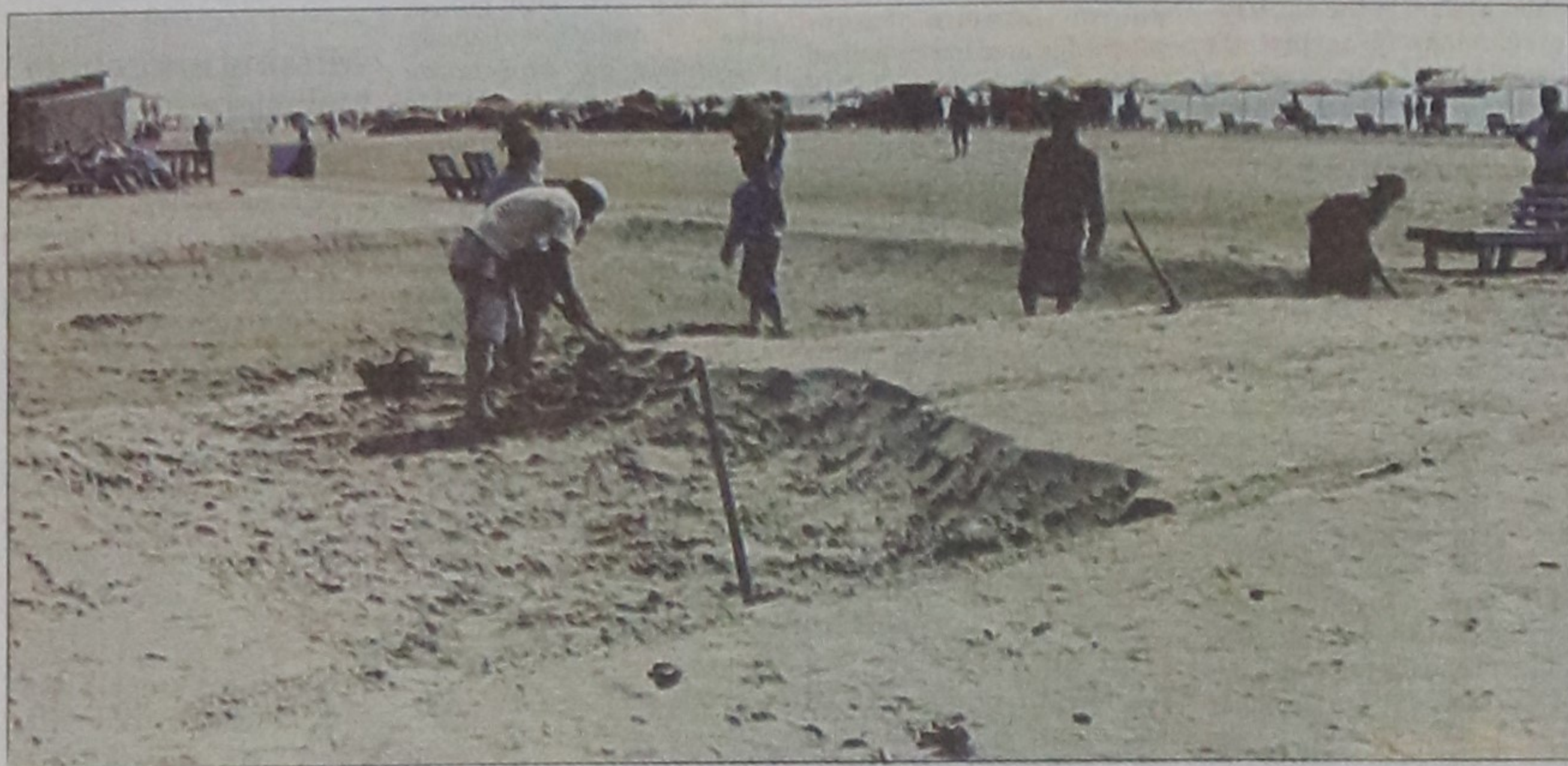
Sand lifting on Kuakata sea beach, being done to repair an LGED rest house nearby, makes the area vulnerable to erosion by waves.
