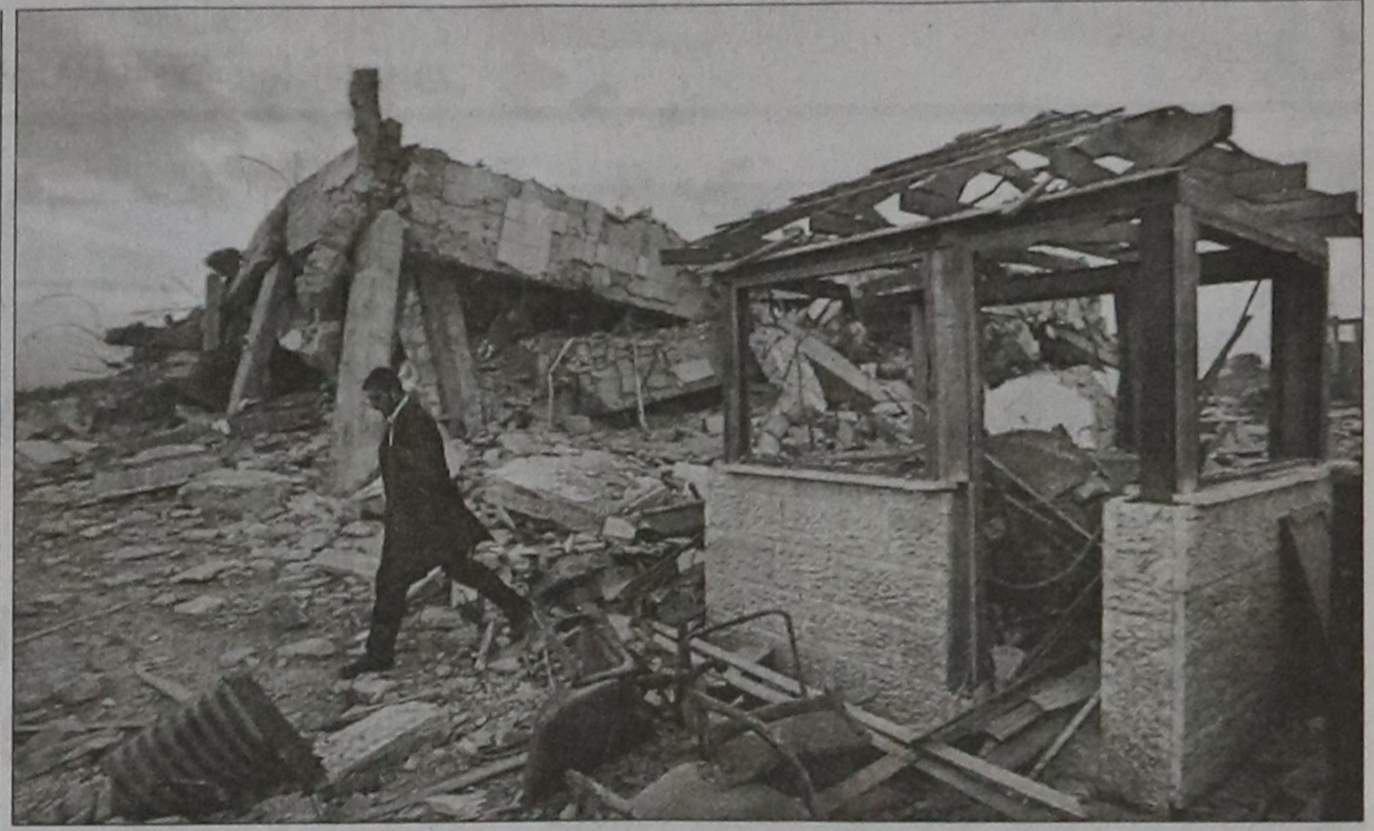
A security member of the Islamic Resistance Movement Hamas walks through rubble of the destroyed presidential offices in Gaza City on Saturday. Israeli bombing and airstrikes razed virtually the whole compound during the 22-day assault on the Gaza Strip that left 1,300 Palestinians dead before it ended on January 18.
