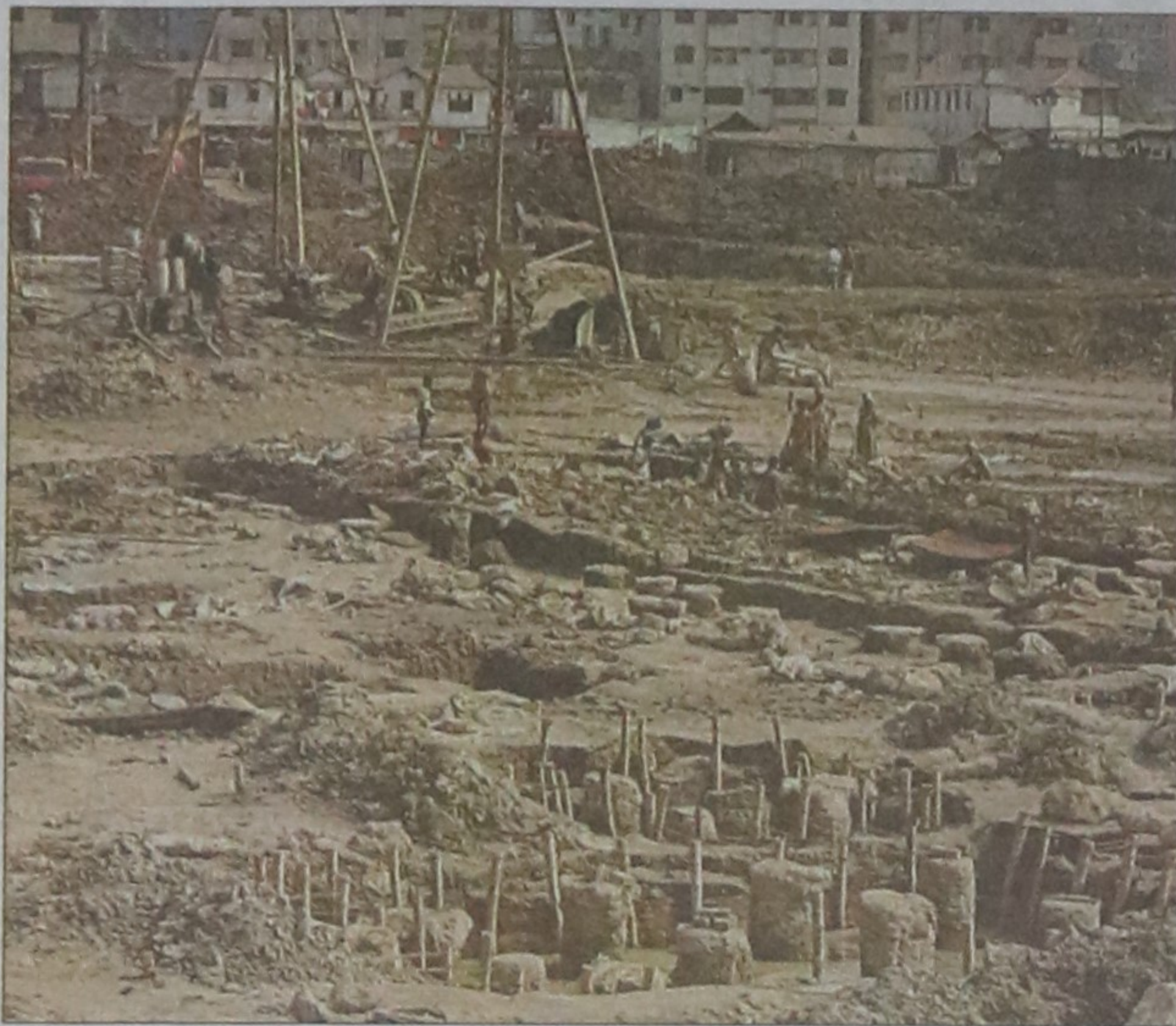
Construction of the kitchen market in progress at Mahakhali.
