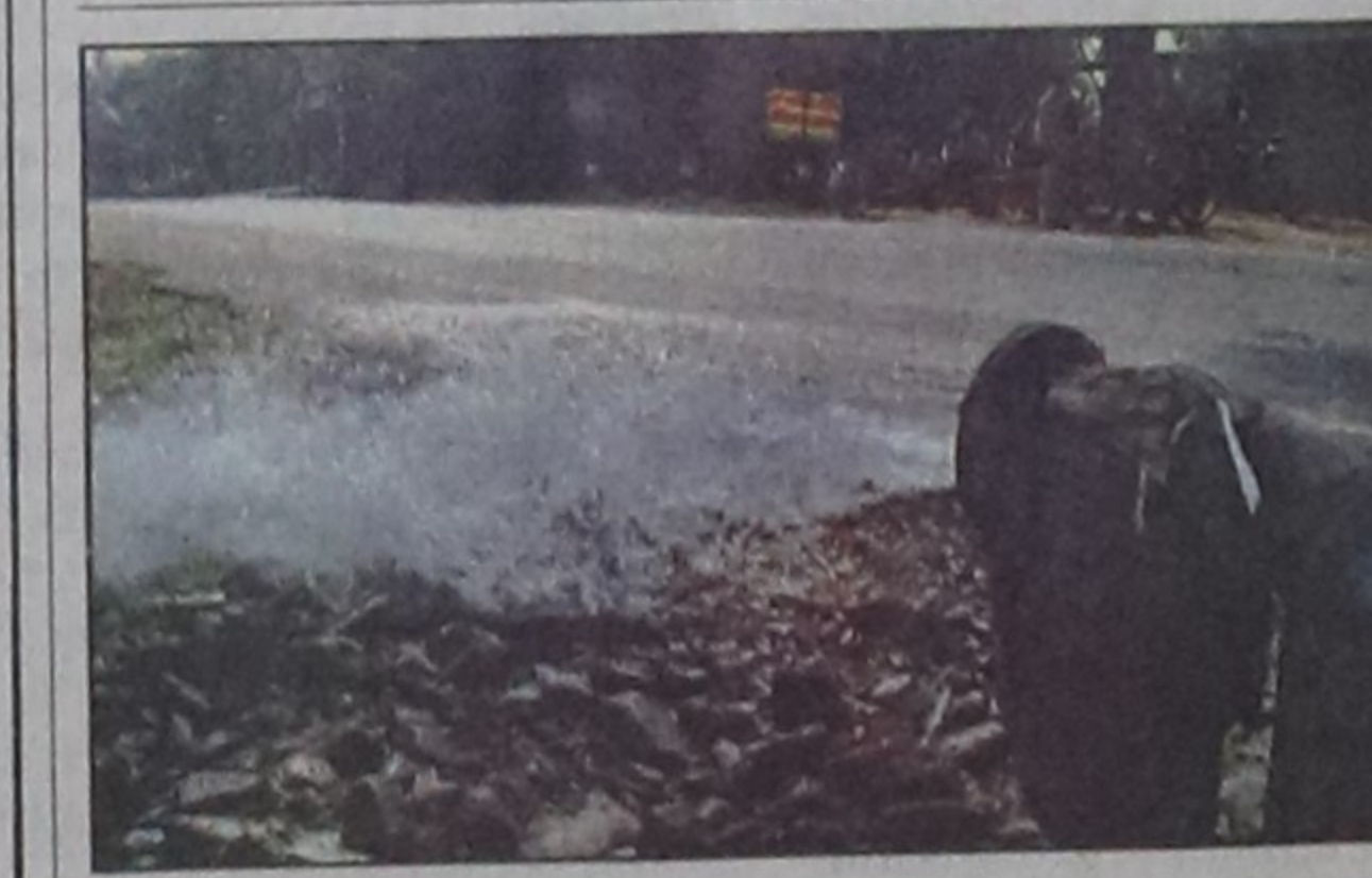
This supply line in Naohata pousava in Rajshahi district has continued wasting water for six months, thanks to authorities' indifference.
