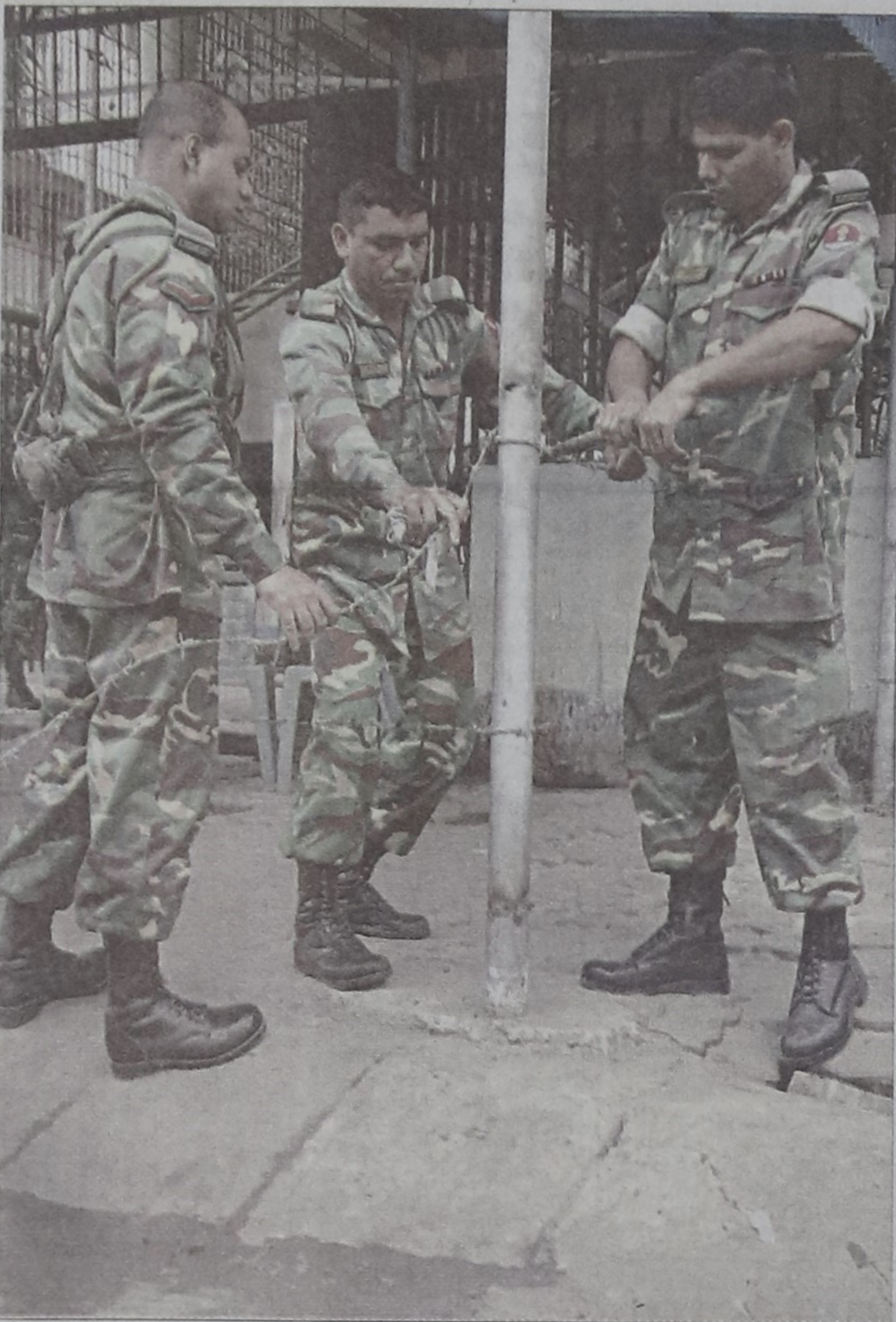
Army personnel yesterday set up barbed wire fences at Paltan Community Centre as they turn it into a temporary camp. The army will be deployed today across the country to ensure security during the upcoming elections.
