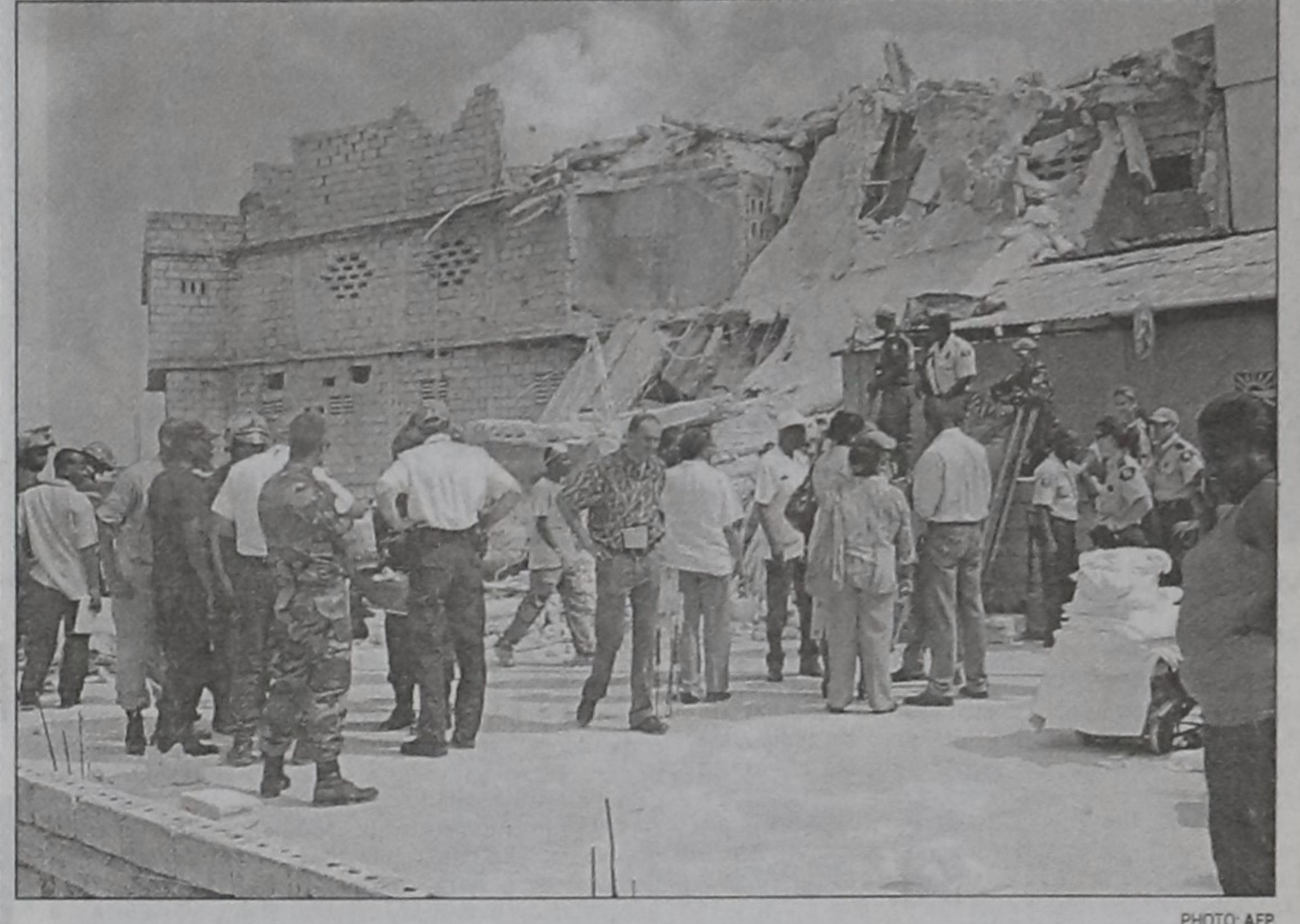
Picture shows people gathered at the site of the collapsed College Promesse Evangelique at Petion-ville in Haiti yesterday.
