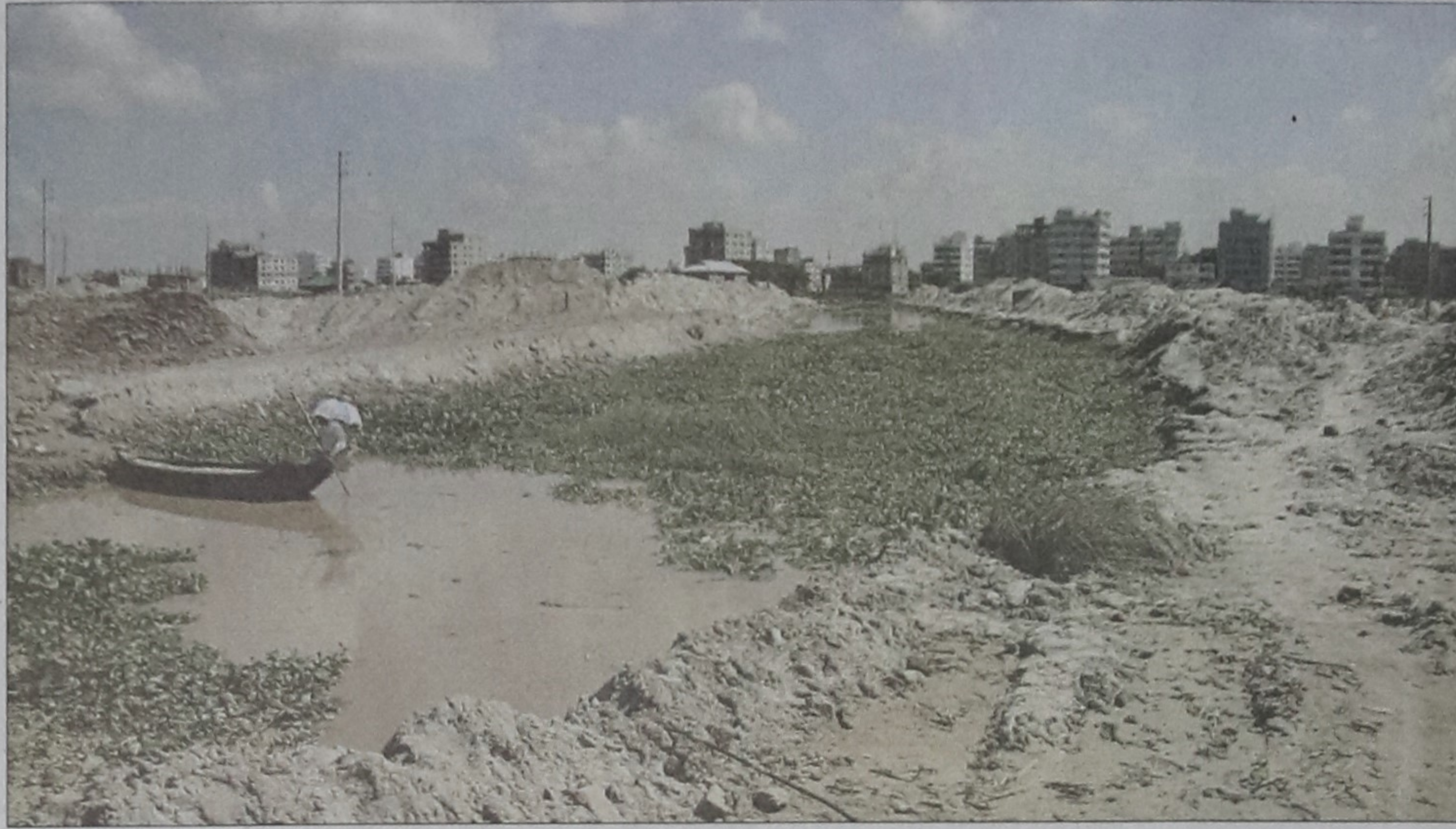
Recovery drive gets tough in Sutibhola canal in Badda, as a private housing company has already filled part of it with earth and erected quite a few concrete structures.
