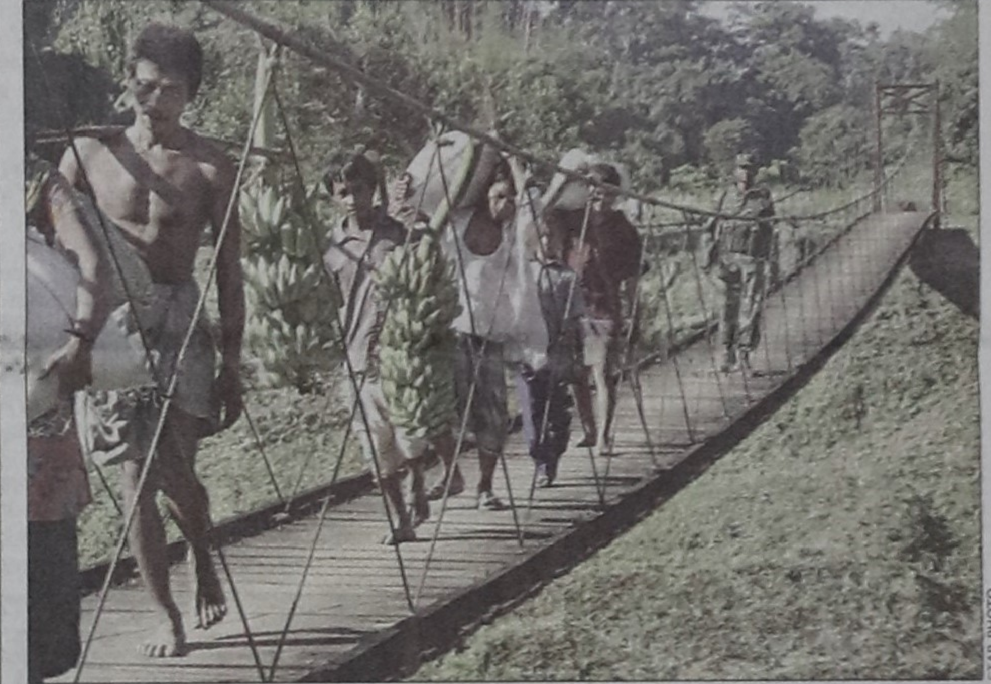
Indigenous people cross over the hanging bridge constructed by the Bangladesh Army (Matiranga zone) on the Toimathoi Chhara canal at Matiranga under Khagrachhari.
