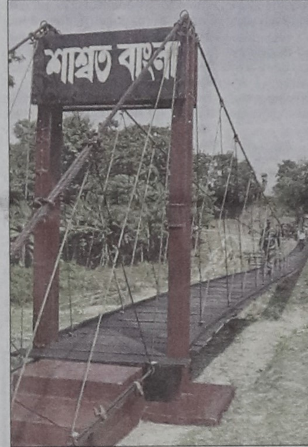
the bridge on October 22.
