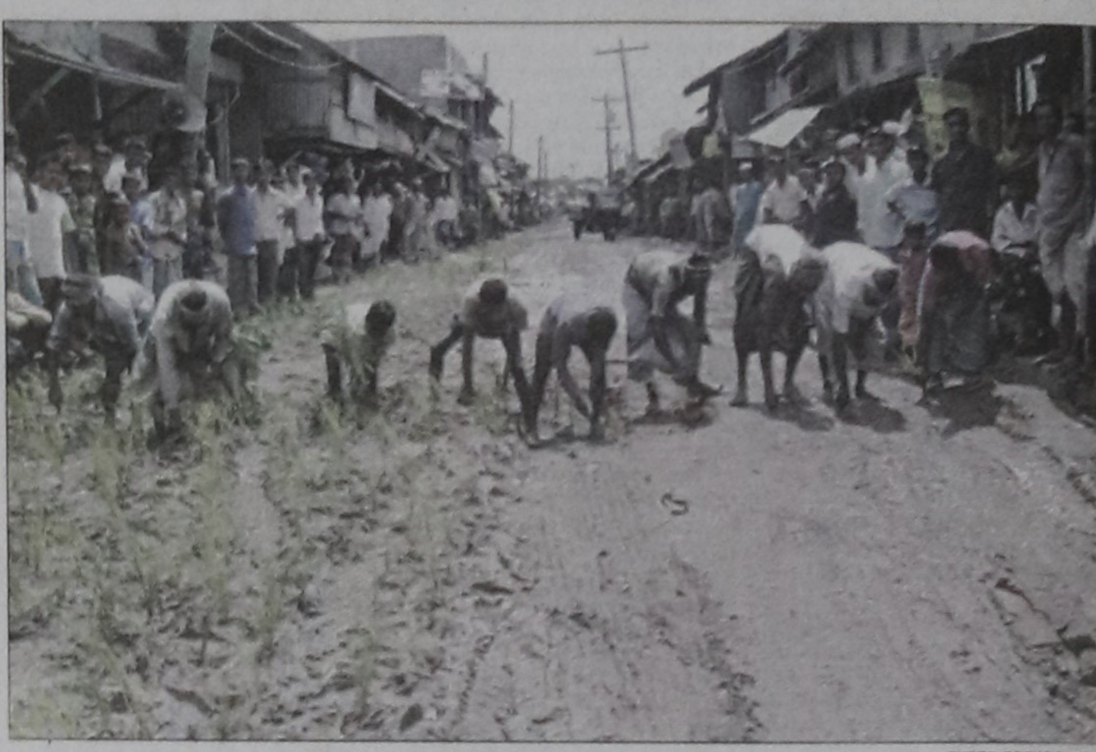
Local residents and traders plant paddy seedlings on the Kolapara-Kuwakata road in a unique protest against the authorities' negligence in repairing this dilapidated road.
