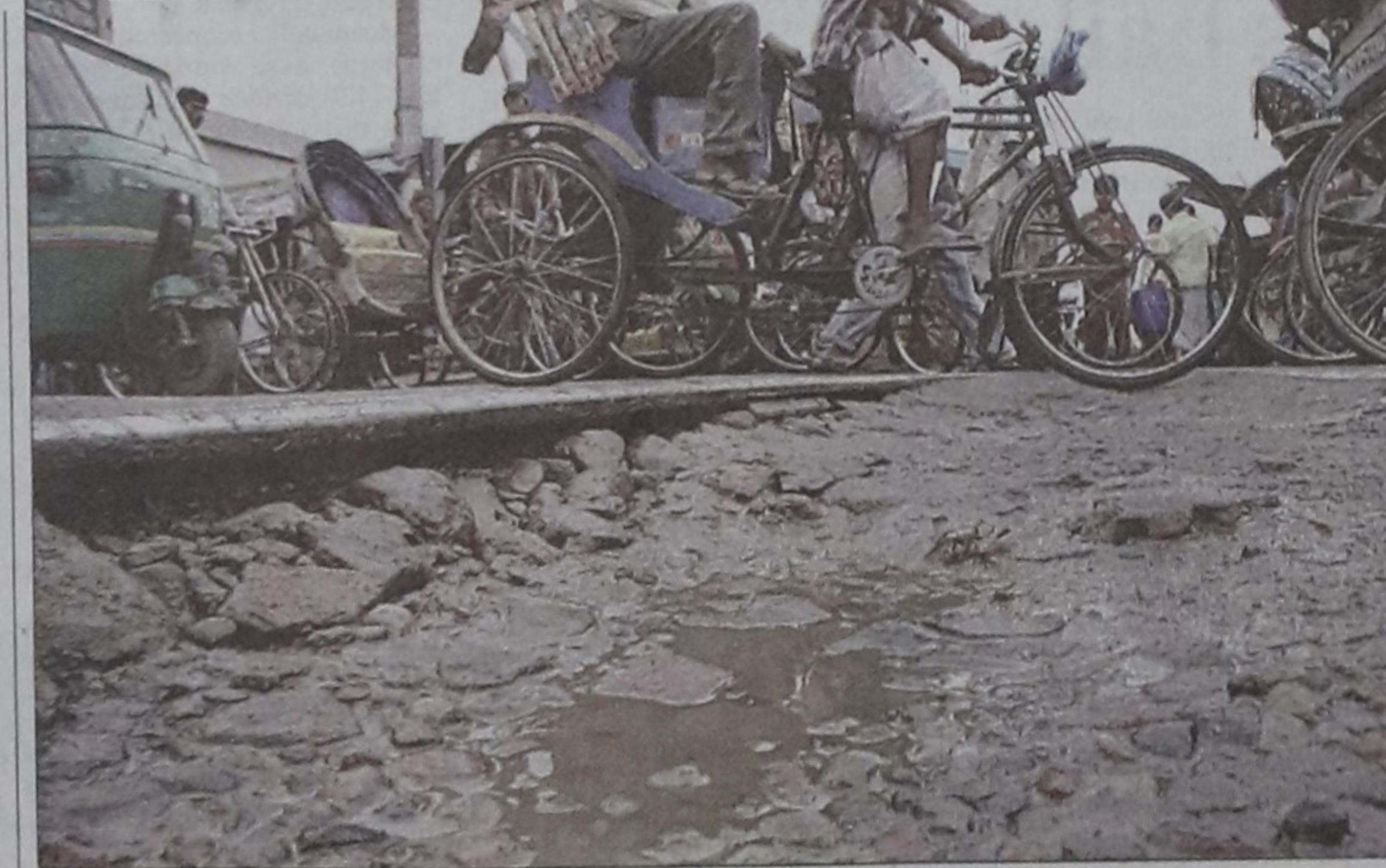
People especially rickshaw riders suffer as the Jurain level crossing in the capital remains in a bad shape with asphalt loosening off the rails due to lack of maintenance.
