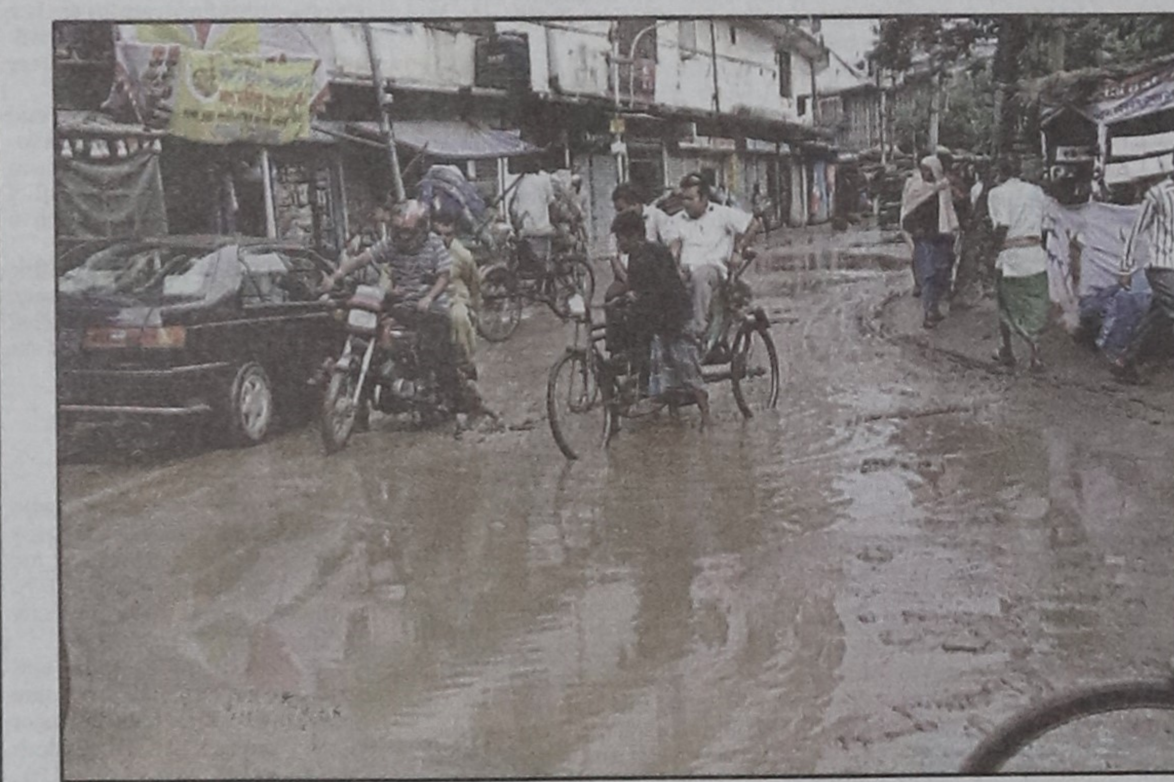
Vehicles negotiate a rundown road in Banshbari of Mohammadpur yesterday. The appalling condition of the road has caused several accidents.
