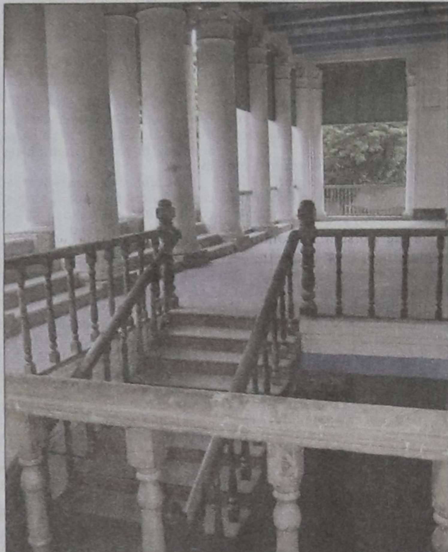
The wooden staircase leading to the pillared veranda with joist and parline roof on the first floor of Pogose School.
