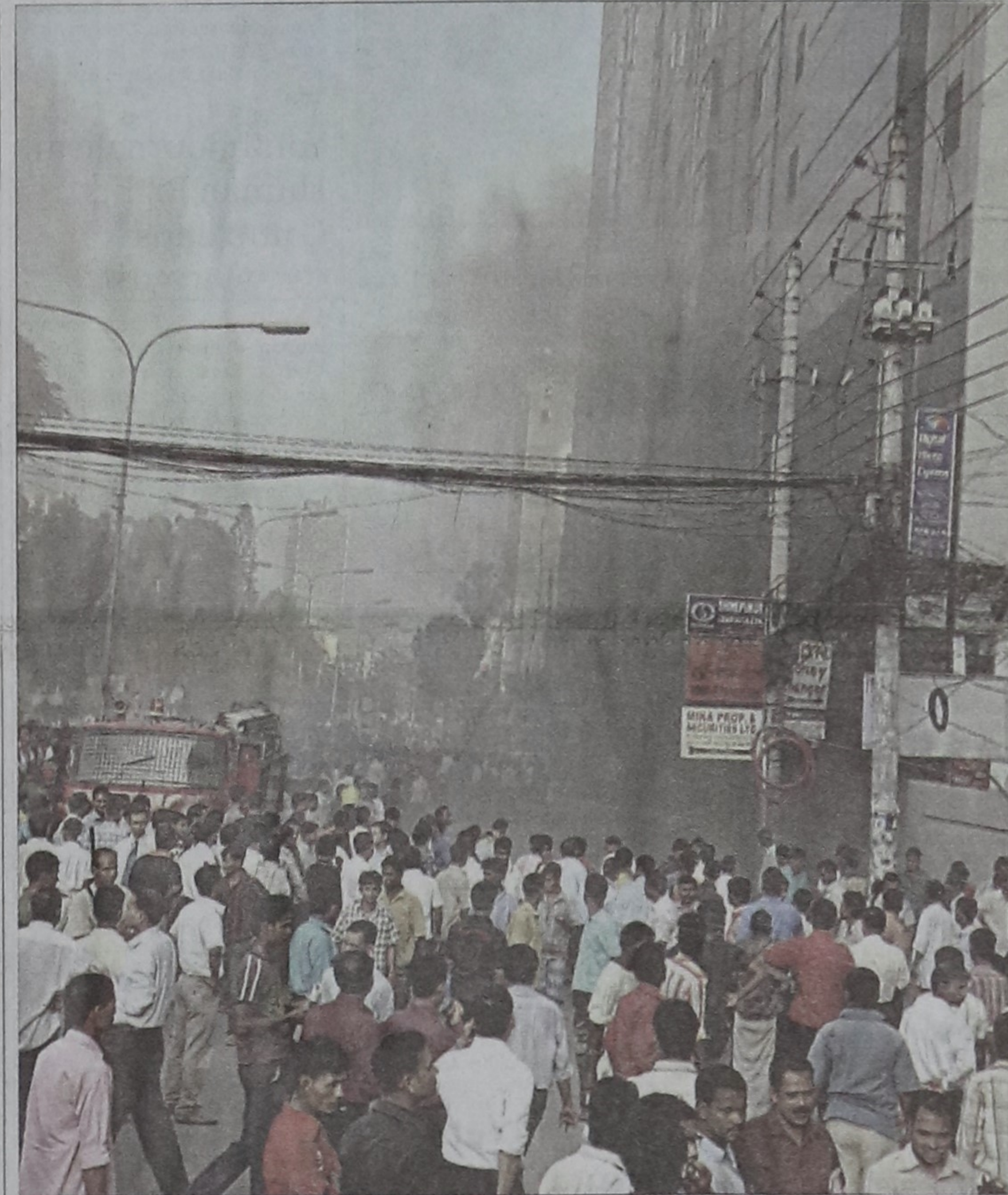
Smoke engulfs 23-storey Faruk Rupayan Tower at Banani in the capital yesterday after a car catches fire at its basement.
