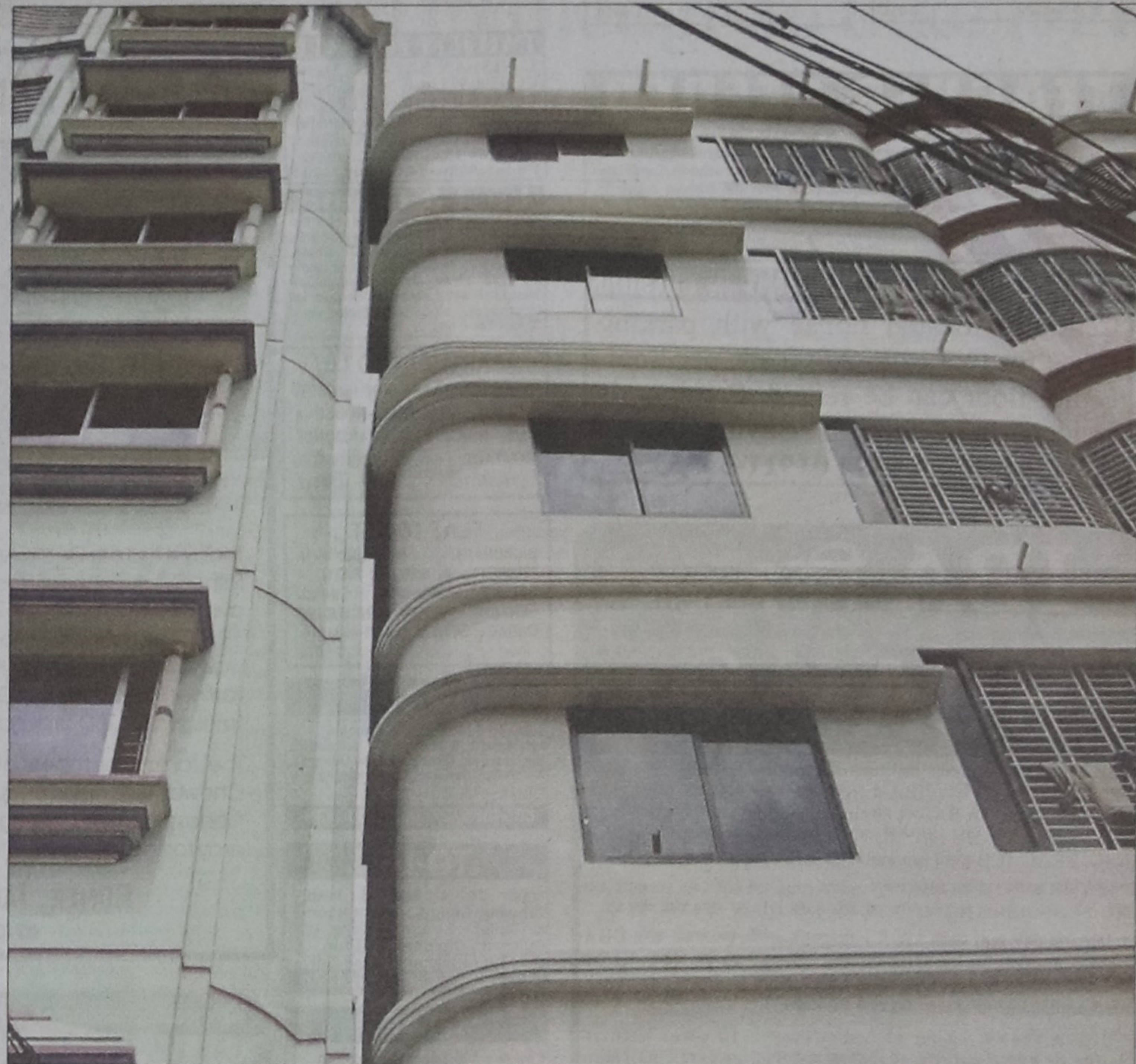
Haji Bhaban, right, at Masterpara leans on another building following an earthquake that hit Rajshahi on Saturday night.
