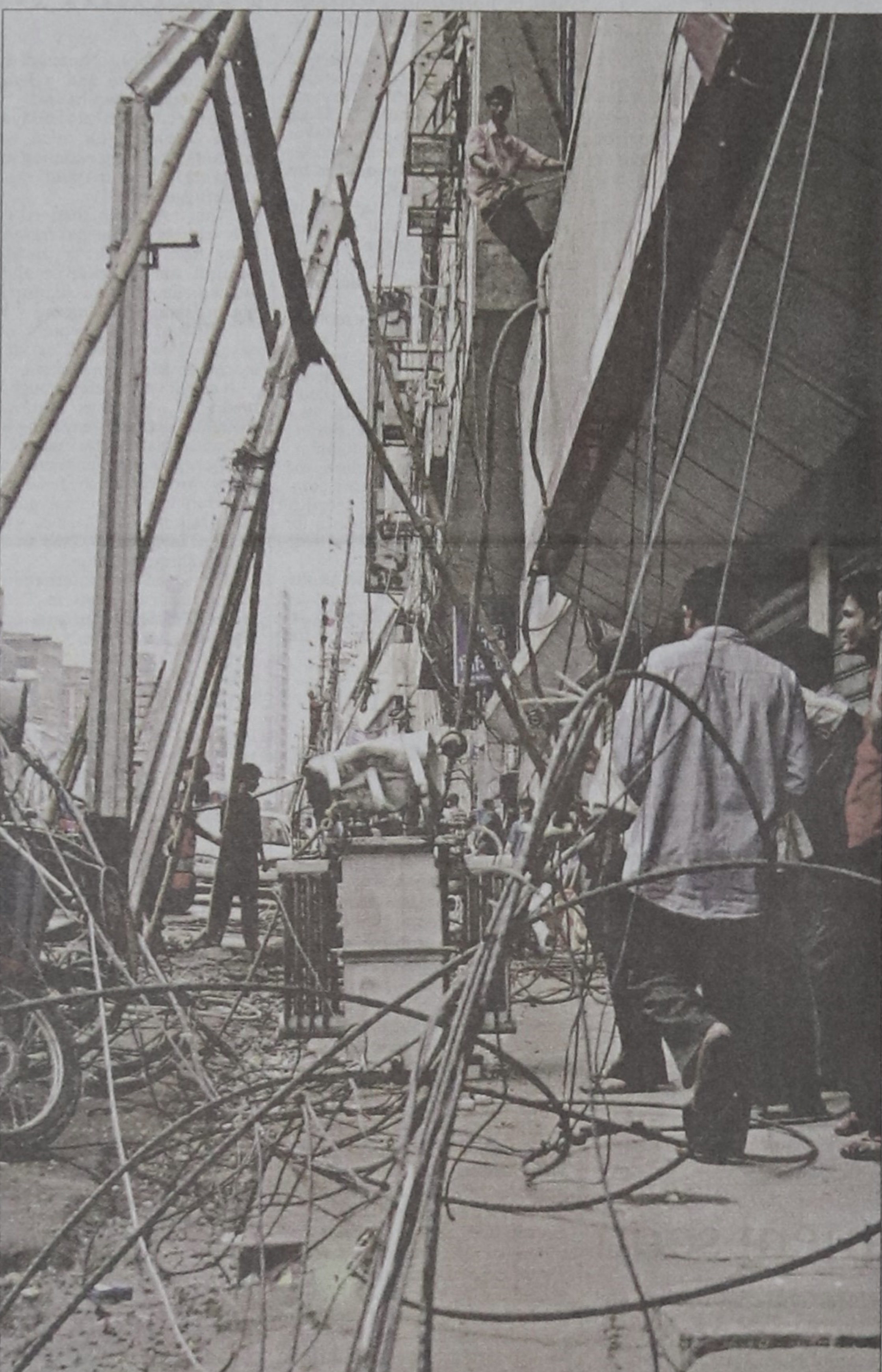
A truck losing control early yesterday rammed the electric poles bearing a transformer in Motijheel in Dhaka. The accident switched off power supply to a number of neighbouring areas.
