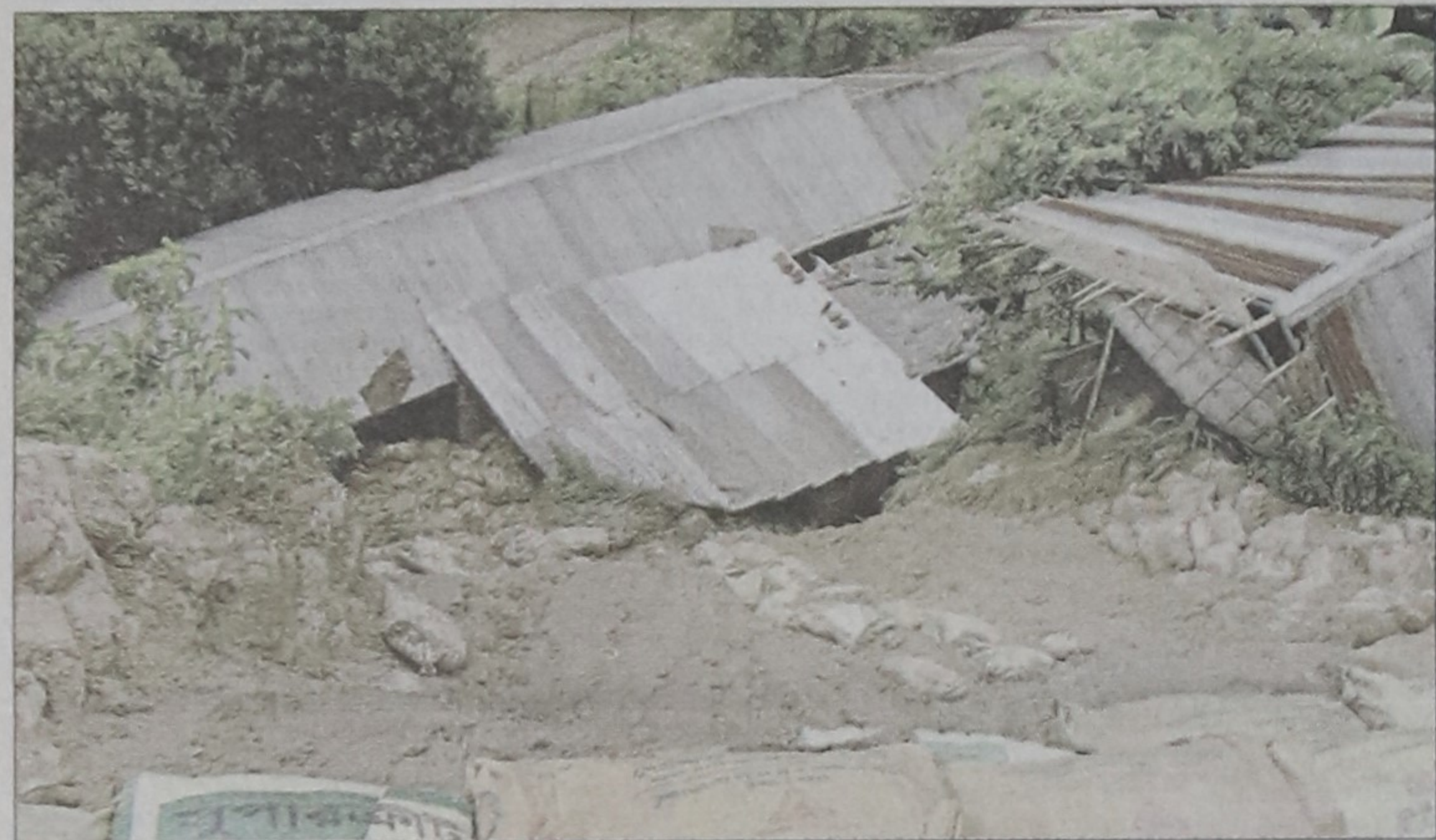
Landslide triggered by incessant rain crushed five houses at Sholoshahar in Chittagong early yesterday. Two people were injured in the incident.
