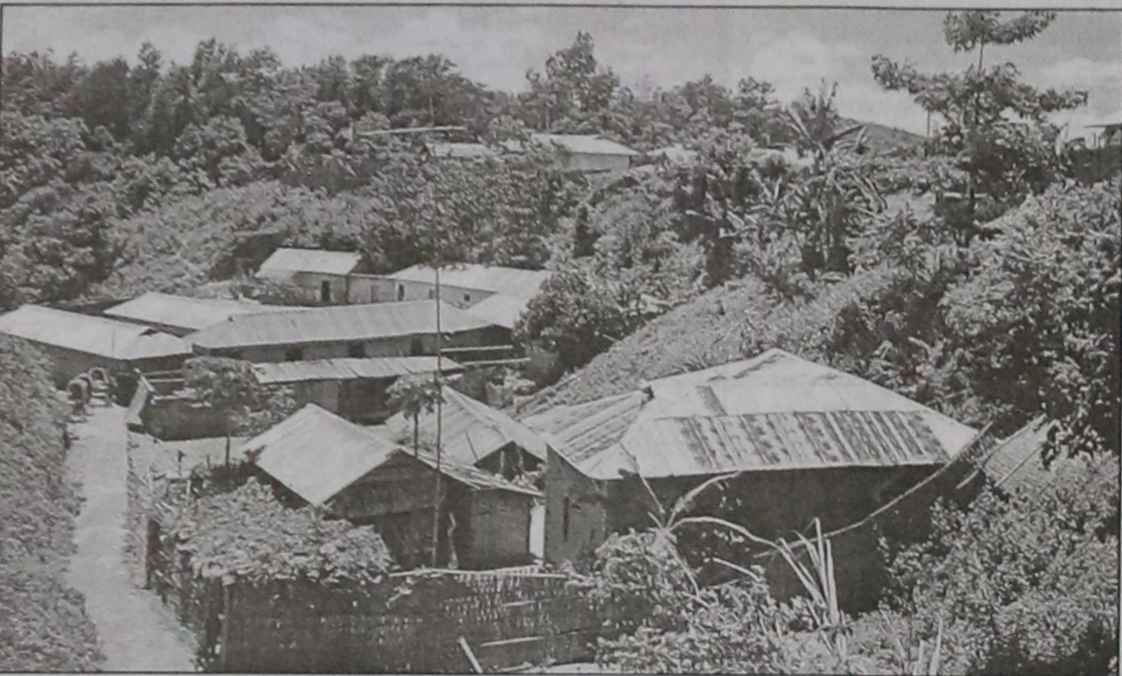
ANGEROUS LIVING ON HILL SLOPES: Homestead built after trimming down hills at Sabujbagh in Sadar upazila in Khagrachhari district poses risk of landslide as the rains have set in.
