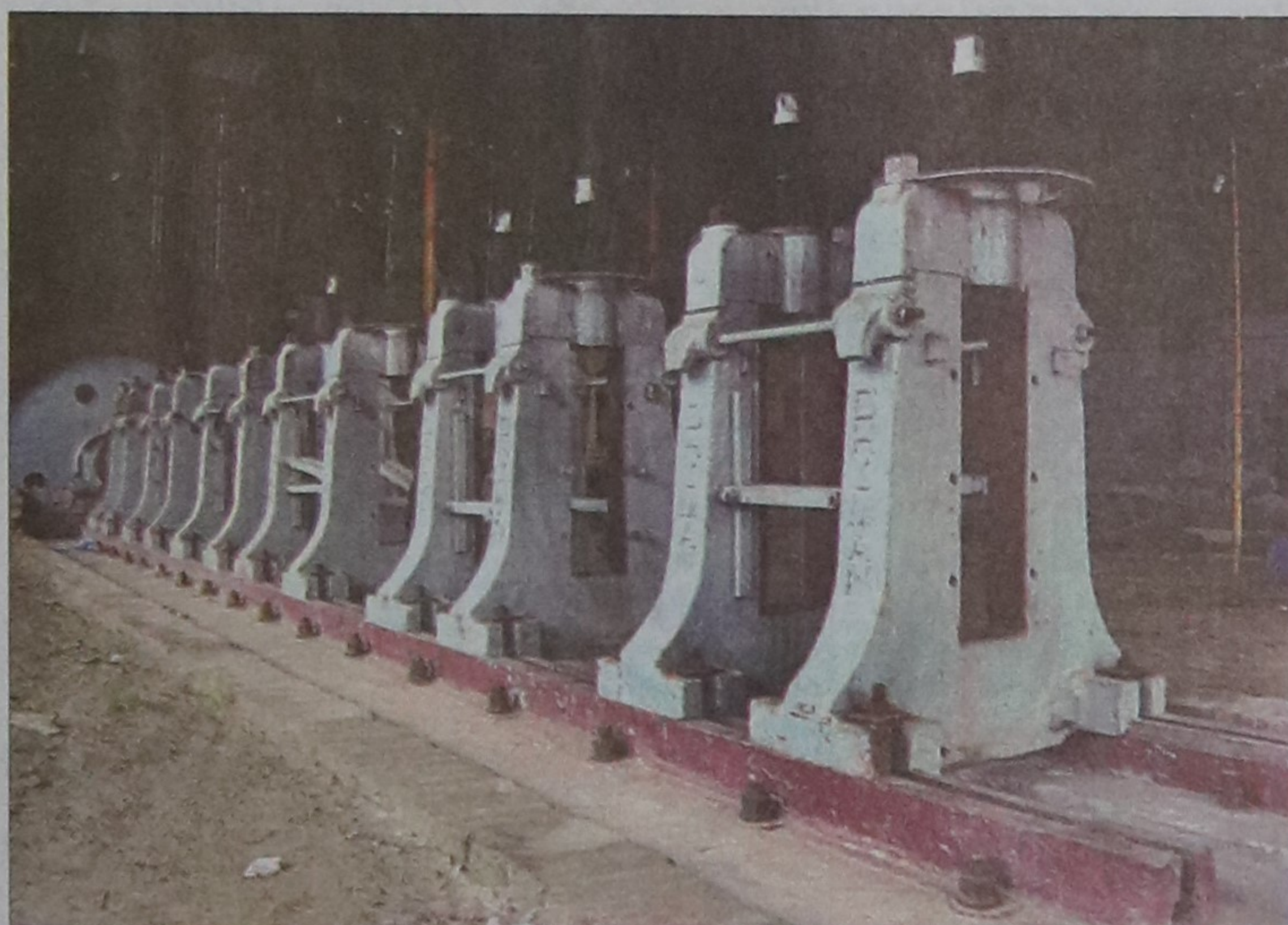
Machinery at Pragoti Steel Mills Ltd lies idle due to absence of gas connection.
