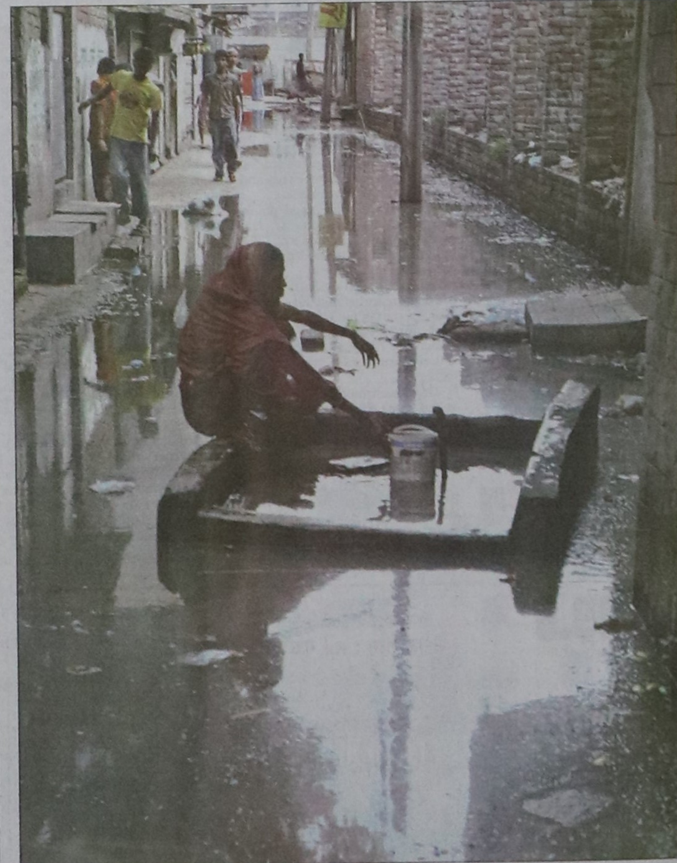
The photograph itself is enough to tell the tale of this lane at Rahmatganj under Ward 65. It remains waterlogged for most parts of the year due to faulty drainage system in the area. The water stands knee-deep just after a downpour. The situation did not change for the last five years despite the residents' repeated calls for rescue.
