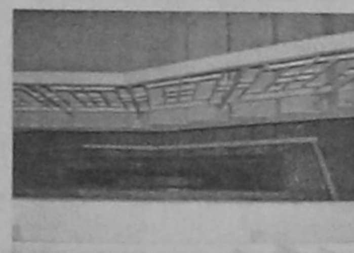
The deadly gap between the flights of a stair
