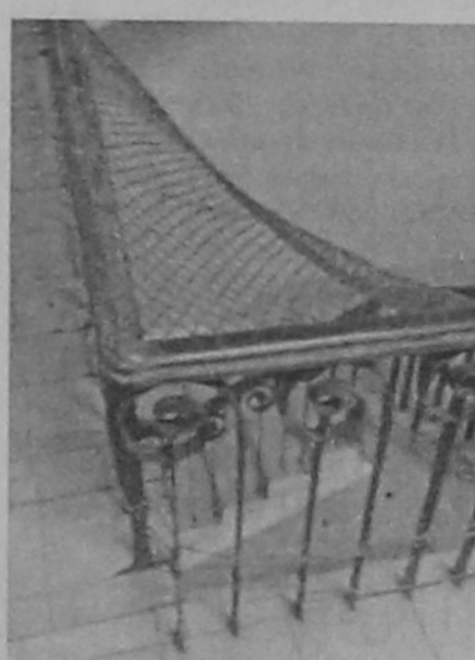
Children may fall victim to even a small gap between the flights of a stair
