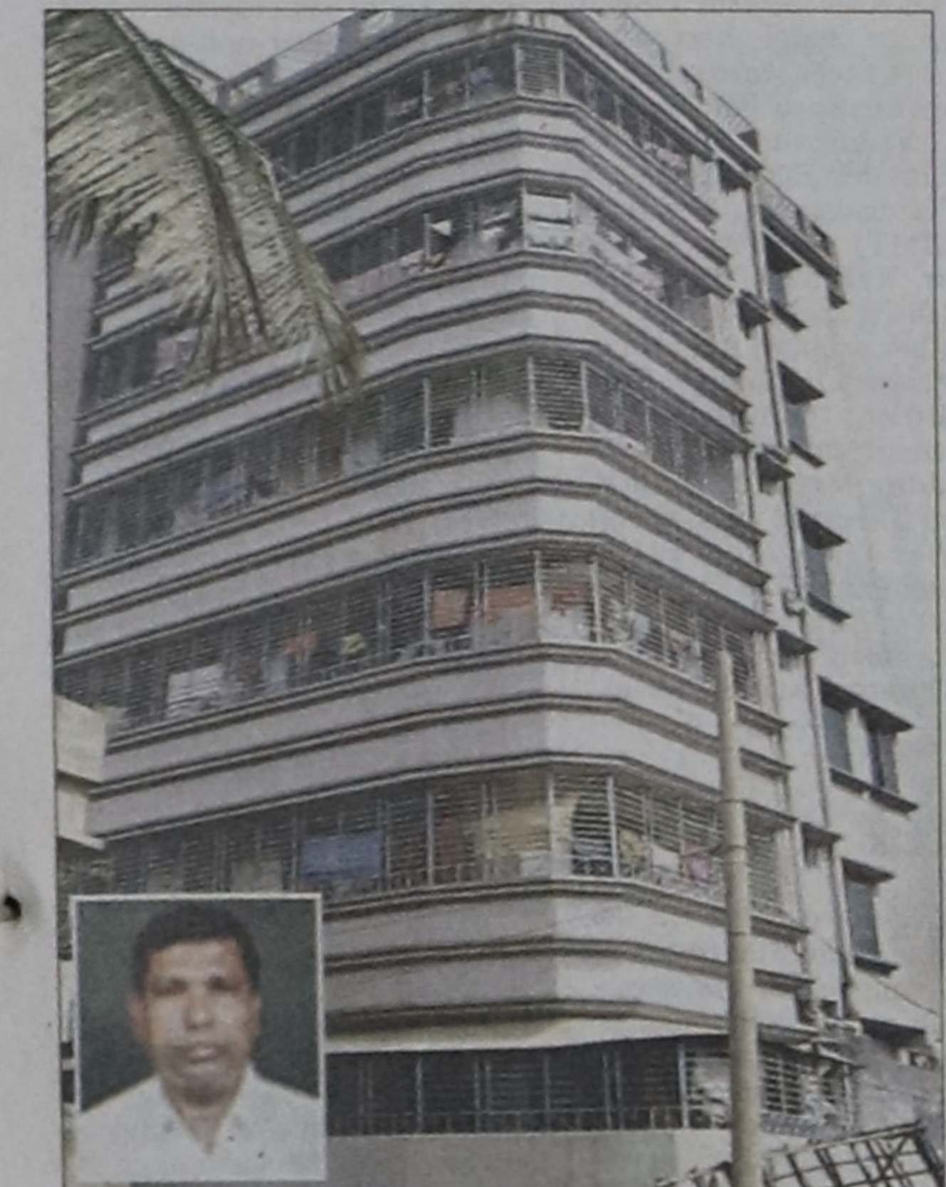
Kafil Uddin Patwari, a third-class employee of Dhaka Electric Supply Authority (Desa) owns this six-storey building in city's Madartek-Basabo area.
