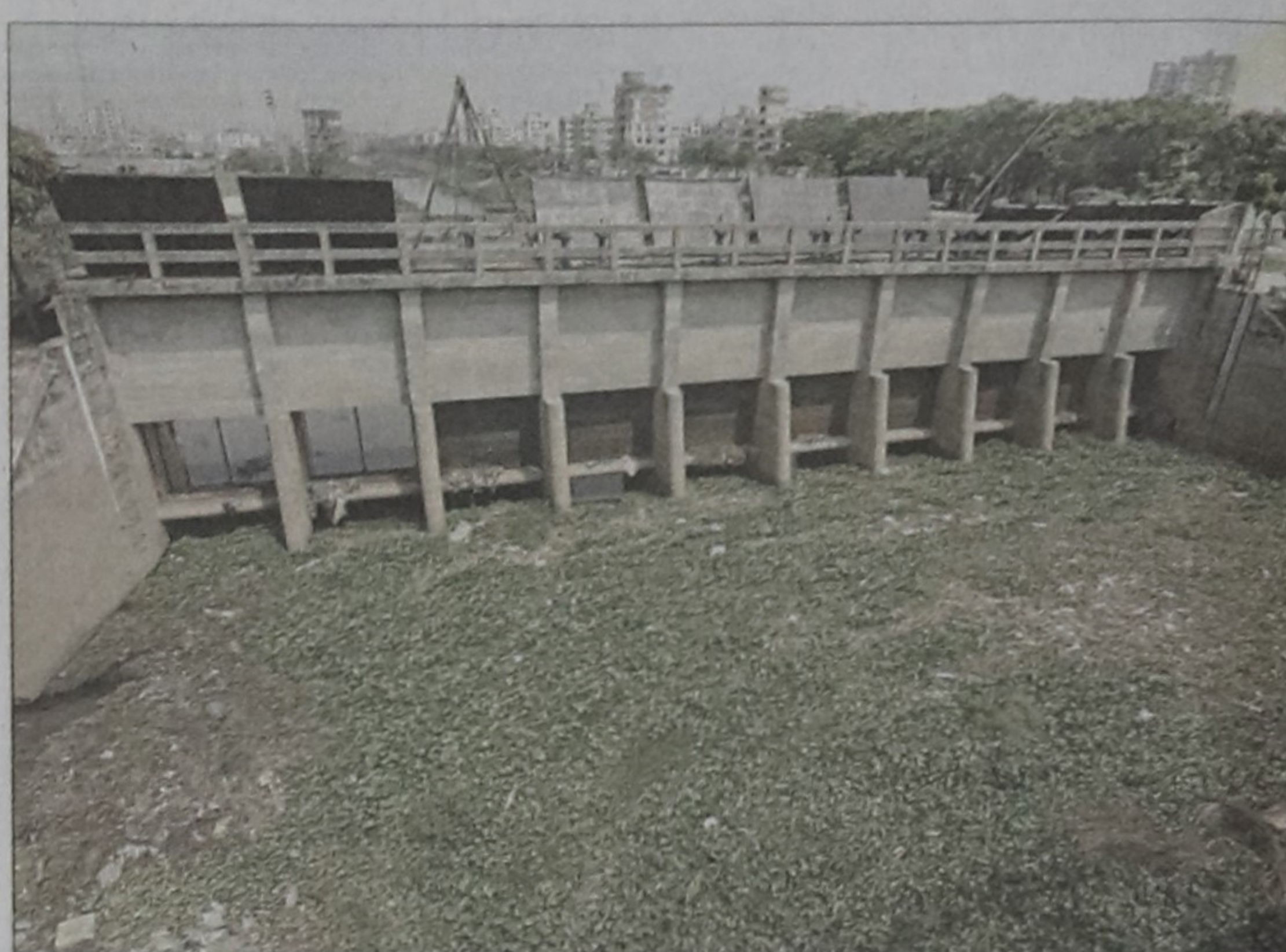
Floating garbage and water hyacinth get stuck at a sluice gate near Rampura Bridge obstructing flow of sewage out of the capital. The photo was taken yesterday.
