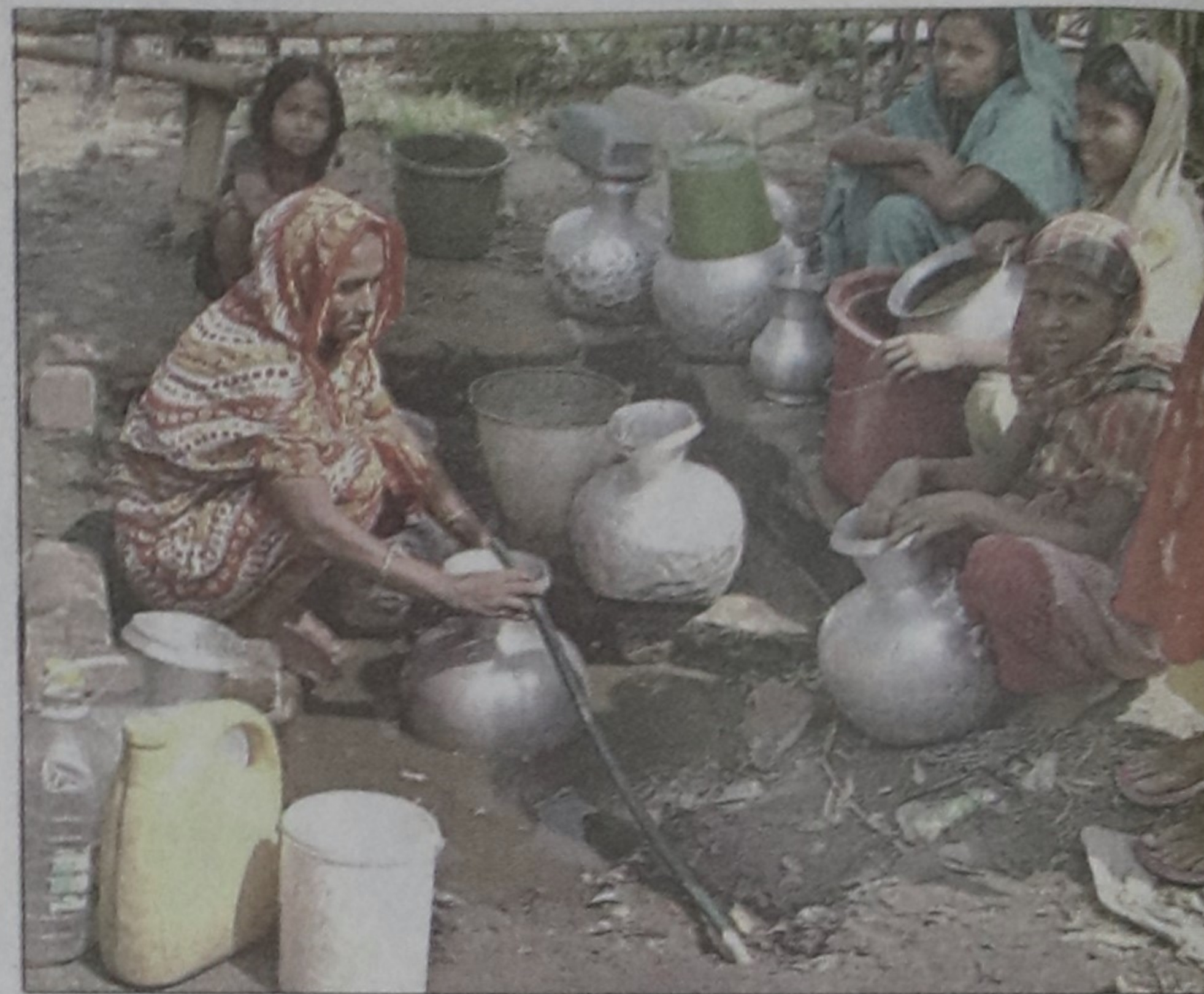
City dwellers in Madarbari area fix a rubber pipe with an underground water line of Wasa to collect water. Women wait in queue for hours for water to be supplied through the pipeline.
